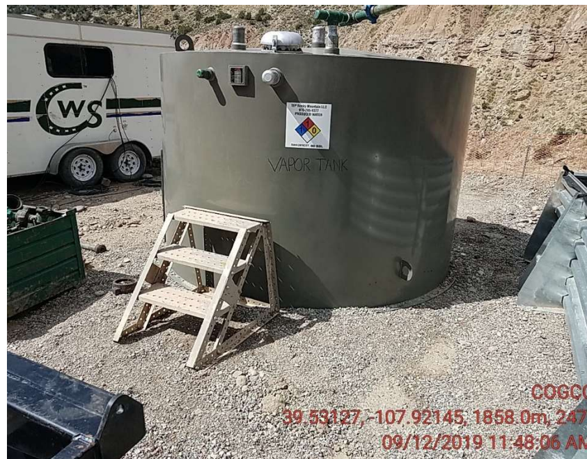
Tank with out secondary containment
