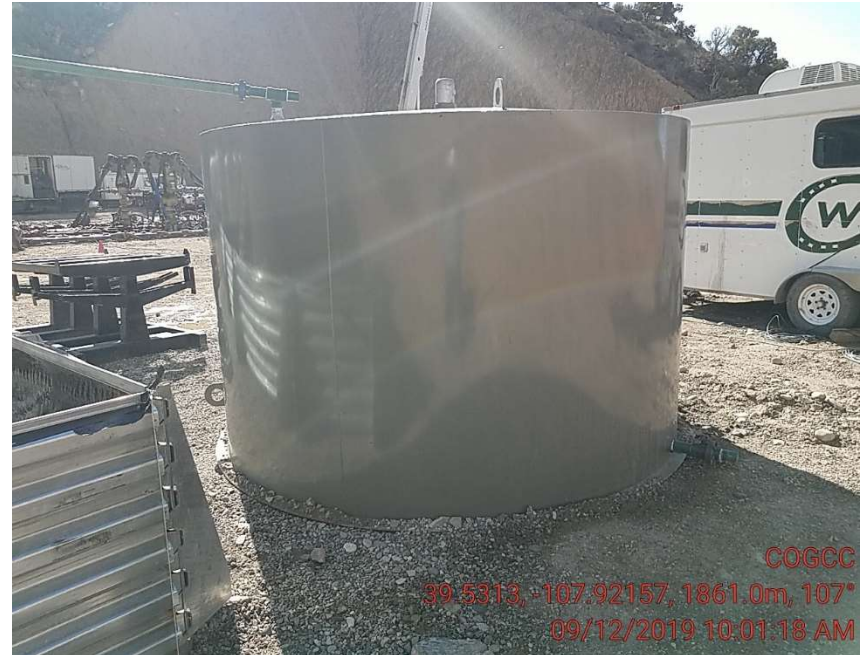
Tank with out secondary containment
