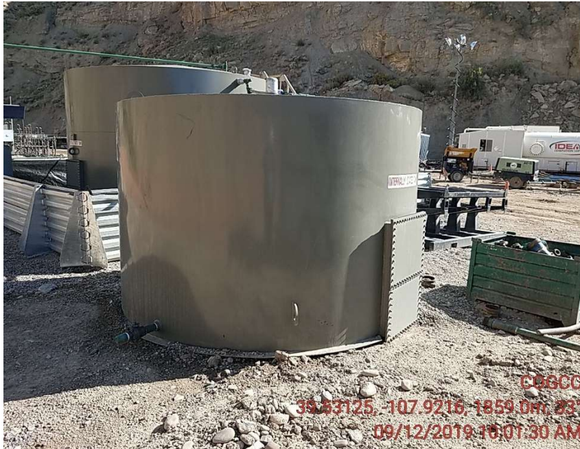
Tank with out secondary containment
