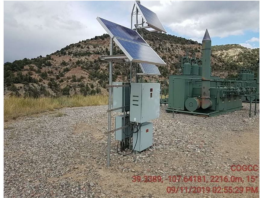
New inspection showing unused equipment is gone.
