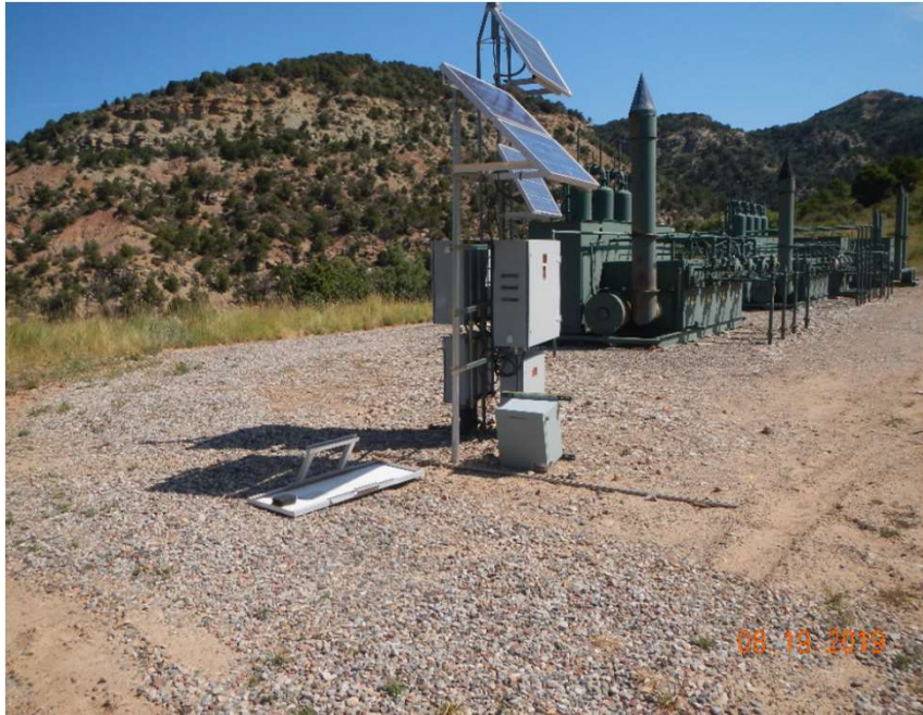
Previous inspection of unused equipment
