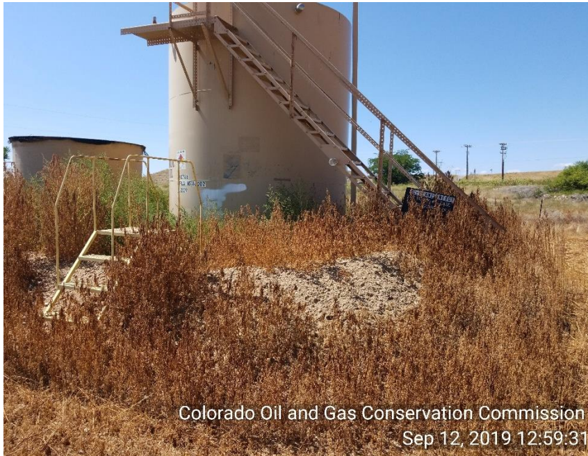
Photo 7 TNK BTRY Sign does not have a working emergency number. WEEDS
