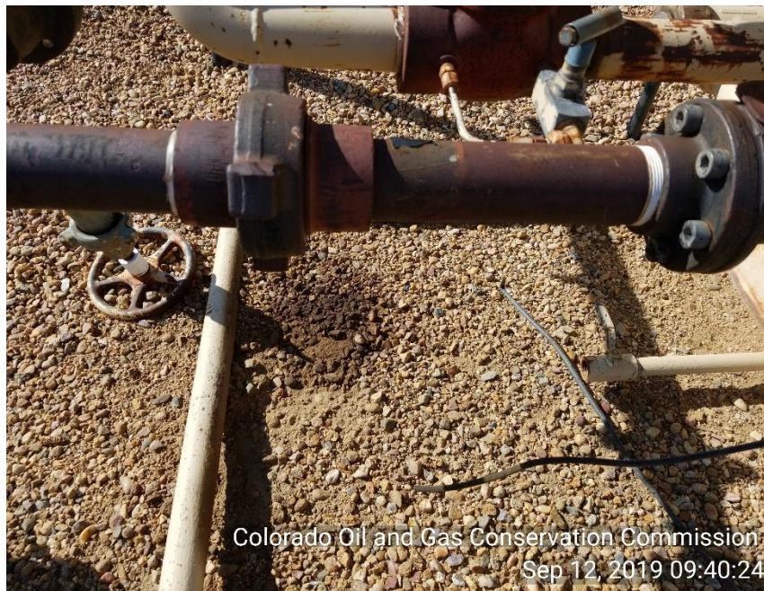
Photo 13 Stained soil under piping out side of separator
