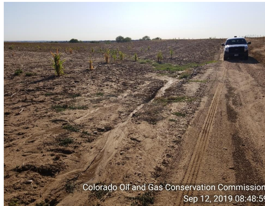
Photo 8 Sediment from erosion on access road being carried off access and into drainage.
