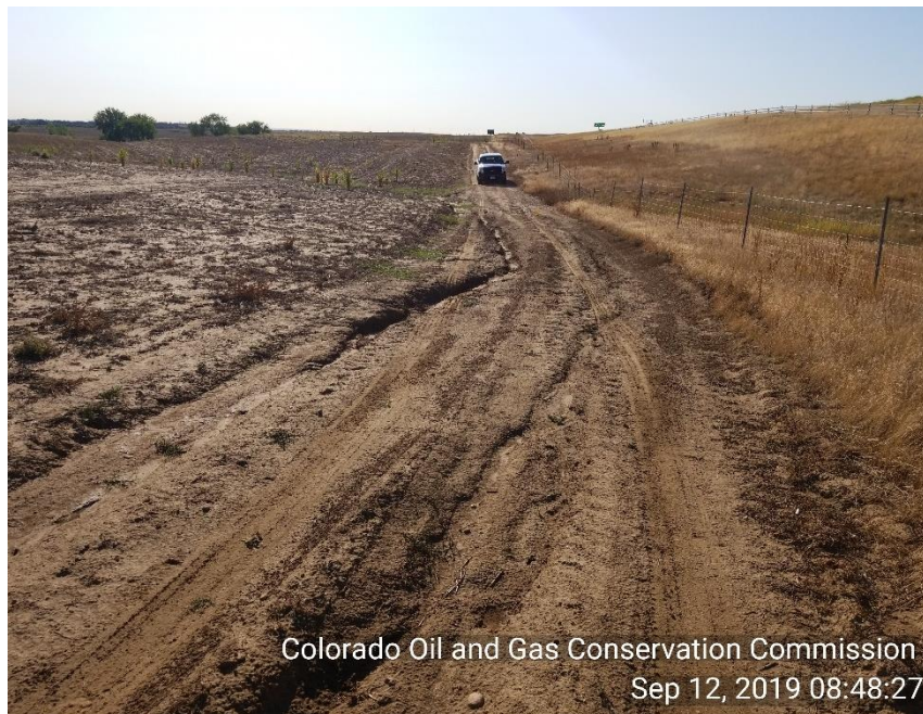
Photo 7 access road to location. Deep ruts and erosion in road.
