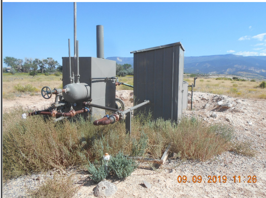
Meter housing and Separator looking NE Weeds. 2" flowline riser w/ plug.
