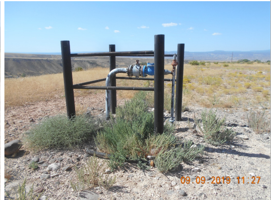
2"x 4" gather line riser w/ pipe barricade. LO/TO. Looking SW Weeds
