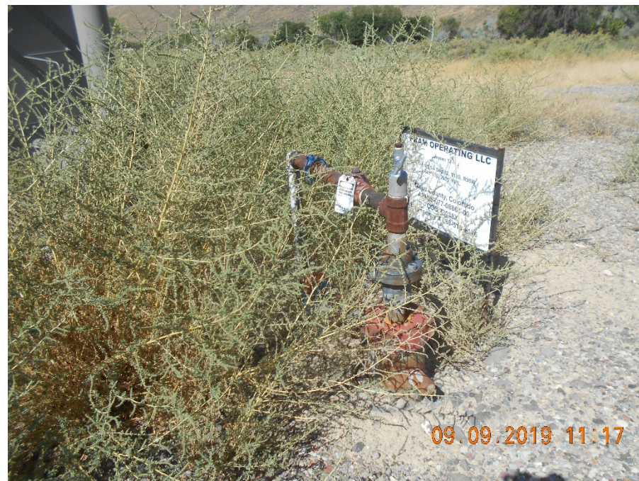
Wellhead with sign. Locked out / tagged out. Weeds
