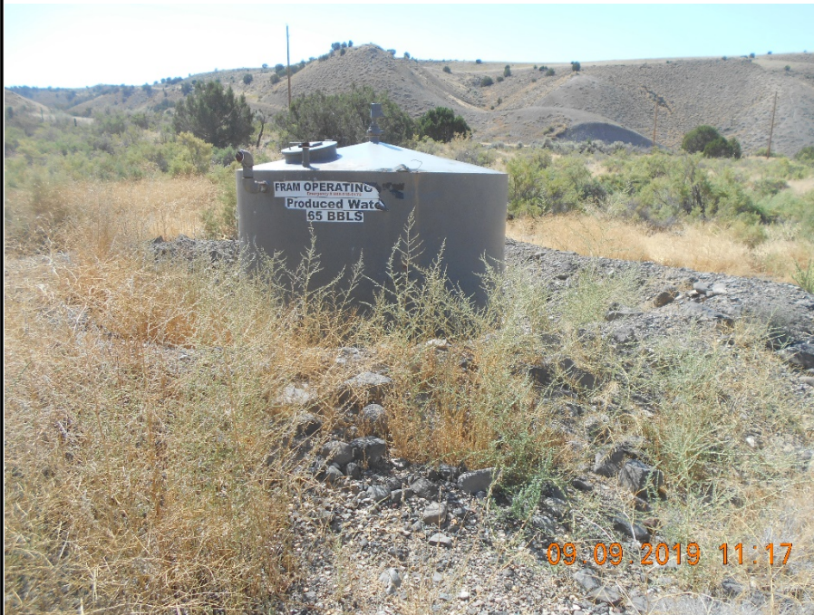
Tank with earth berms looking SE. Disconncted riser with plug at base of tank Weeds
