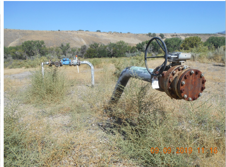
8" gathering line riser. Locked out/tagged out w/ blinde flange. 2"x 4" gather line riser in background. LO/TO.
