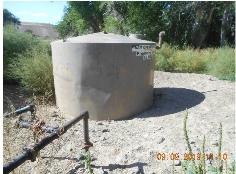
Tank (Disconnected). Berms inadequate. Weeds
