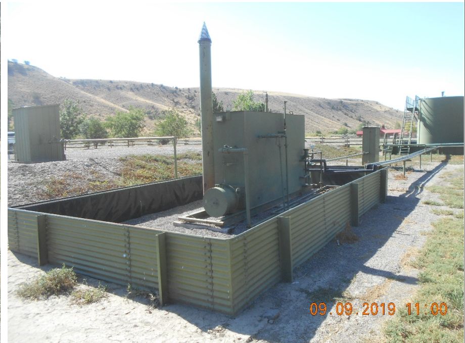
Separator with metal berms. NW corner of berm Looking SE.
