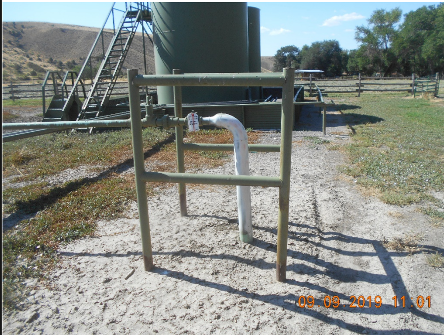
4" gathering line riser. Locked out/tagged out. Pipe barricade.
