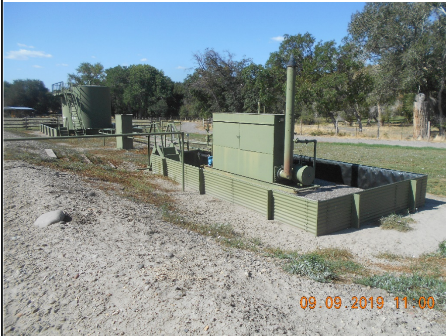
Separator with metal berms. NE corner of berm Looking SW.
