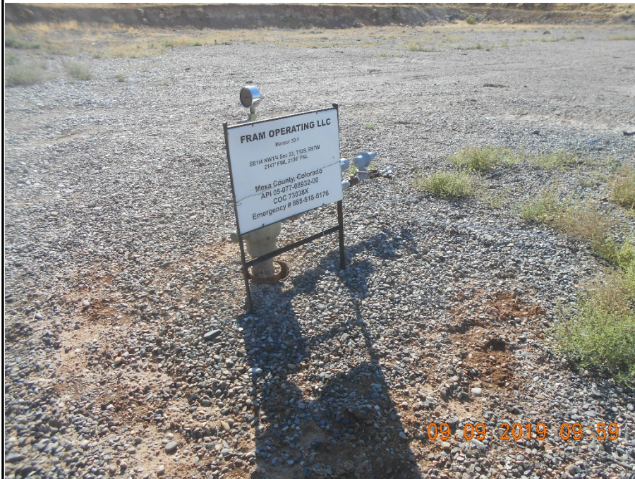
API # 05-077-08932 Mansur 33-1 wellhead with sign. Temporarily Abandoned. 800 psi on tubing gauge.
