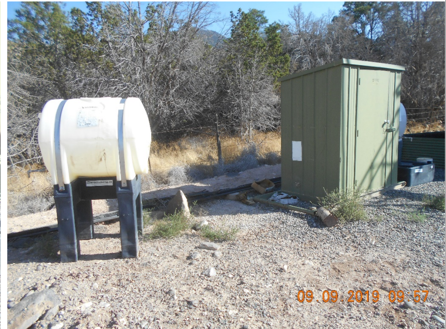
Unused chemical tank without containment on west side of meter housing.
