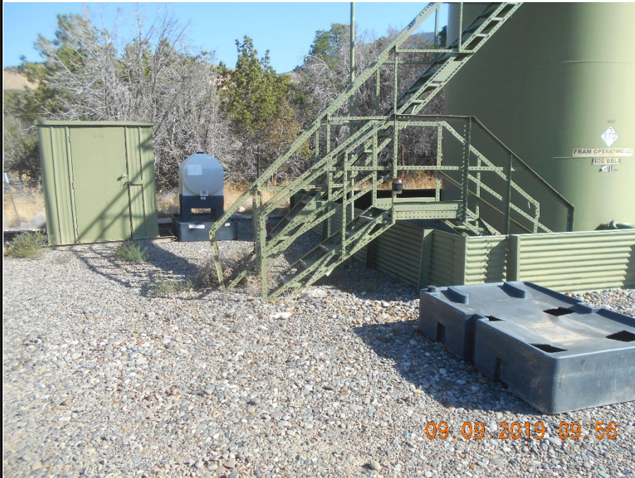
Meter housing on west side of tank battery. Unused chemical injector tank and chemical tank containment.
