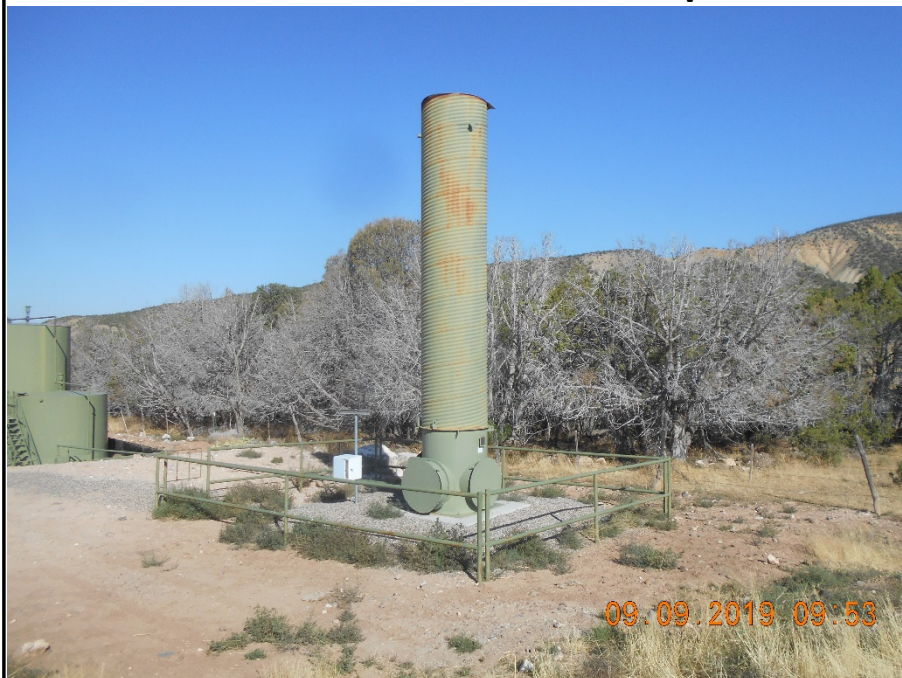
Combustor with pipe fence. Weeds.
