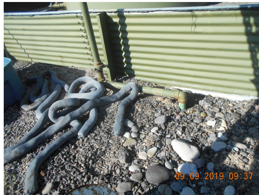
2" Production riser to tank. Located on NE corner of tank battery. Spill response materials scattered by vandal. Oil stained soil.
