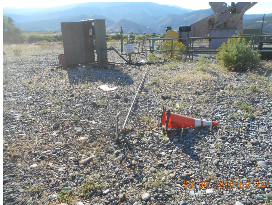
1" flowline riser. Fuel gas supply for 05-077-09326 Seminole 32-2-L pump jack.
