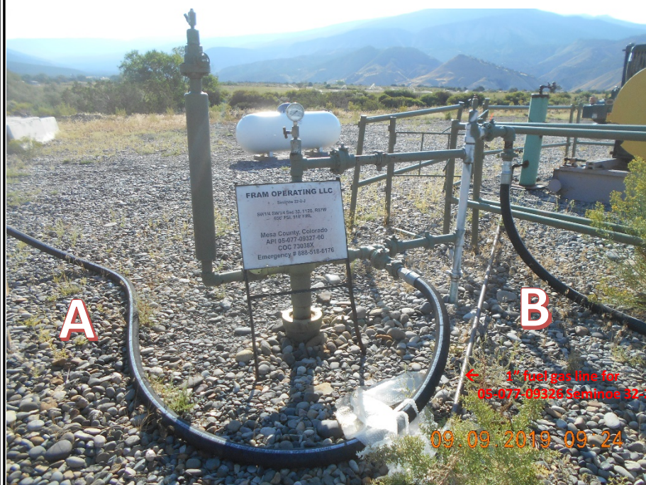
05-077-09327 Seminole 32-2-J. Wellhead with sign. 2" hose connected to wellhead flowing to meter. (A) 2" hose from meter to production riser at wellhead. (B)
