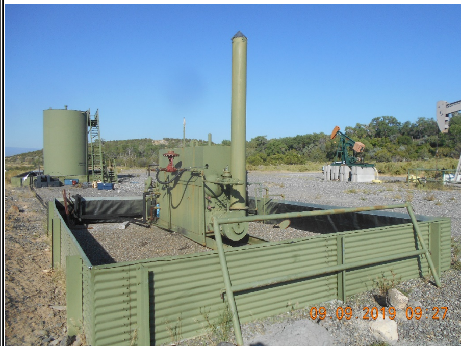
Separator with metal berm. SE corner looking NW. Unused pipe fencing
