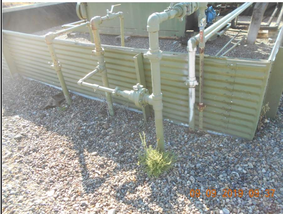
Flowline risers on NW Corner of separator berm. 4x-2" and 1x-1"
