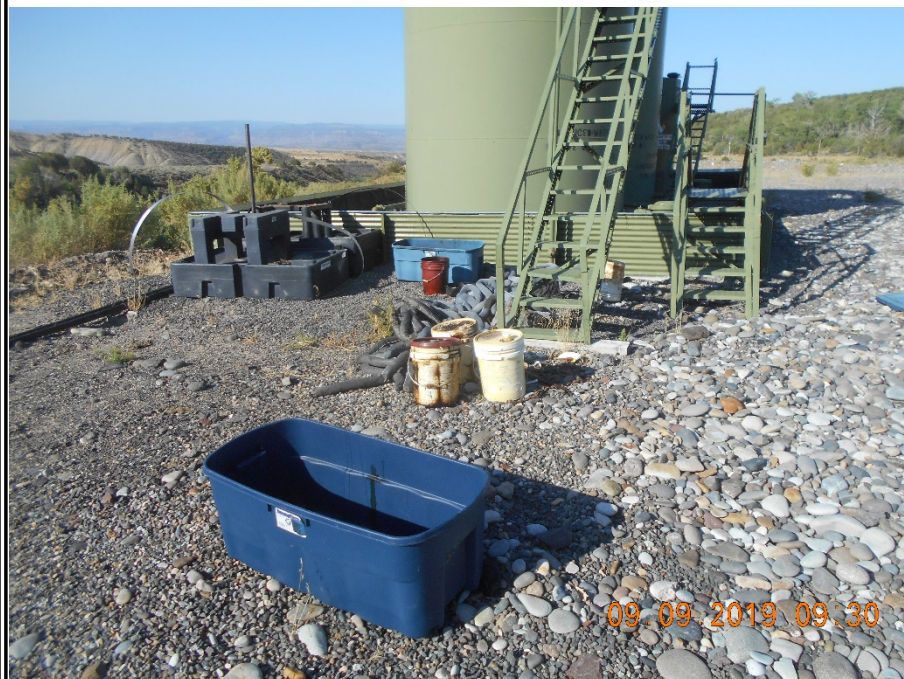
Spill Response Kit materials at E end of tank battery, scattered/stolen by vandals. Injection chemical tank stolen and pump/containment unit vandalized. Oil contaminated buckets and tubs.
