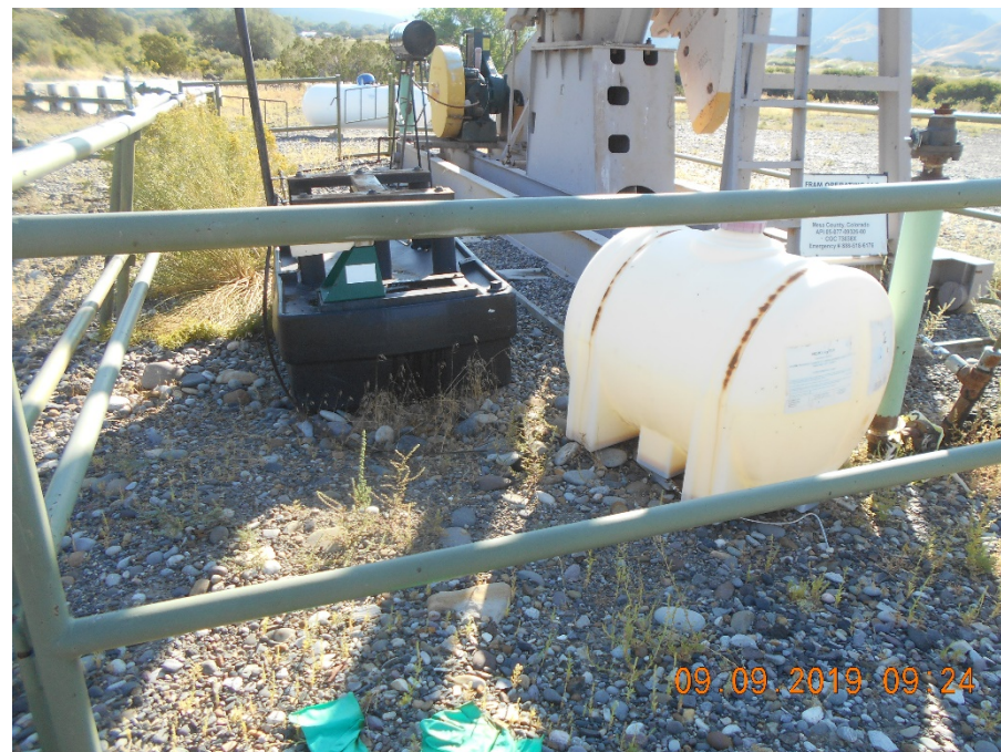
Injection chemical tank and pump/containment unit vandalized. Located at 05-077-09326 Seminoe 32-2-L wellhead
