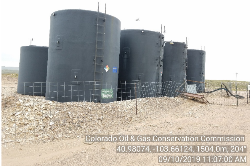
Photo #5 Moyer Unit UIC - Injection Facility Water Tanks
