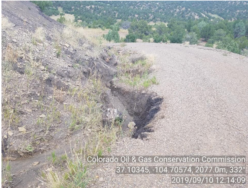
PHOTO 7: EROSION IN BMP DITCH NORTH OF LOCATION. REPAIR EROSION IN DITCH, ADD ADDITIONAL BMP'S TO SLOW STORM WATER FLOW AND PREVENT FURTHER EROSION. COMPLY WITH RULE 1002.f. CA DATE 11-10-19
