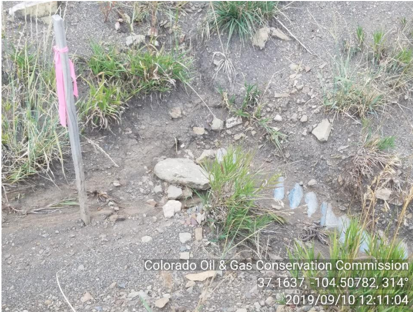
PHOTO 3: CULVERT ON ROW NORTH OF LOCATION IS PLUGGED. CLEAN CULVERT AND PROPERLY MAINTAIN BMP'S, COMPLY WITH RULE 1002.f. CA DATE 11-10-19
