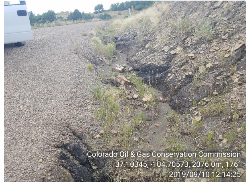
PHOTO 8: EROSION IN BMP DITCH NORTH OF LOCATION. REPAIR EROSION IN DITCH, ADD ADDITIONAL BMP'S TO SLOW STORM WATER FLOW AND PREVENT FURTHER EROSION. COMPLY WITH RULE 1002.f. CA DATE 11-10-19
