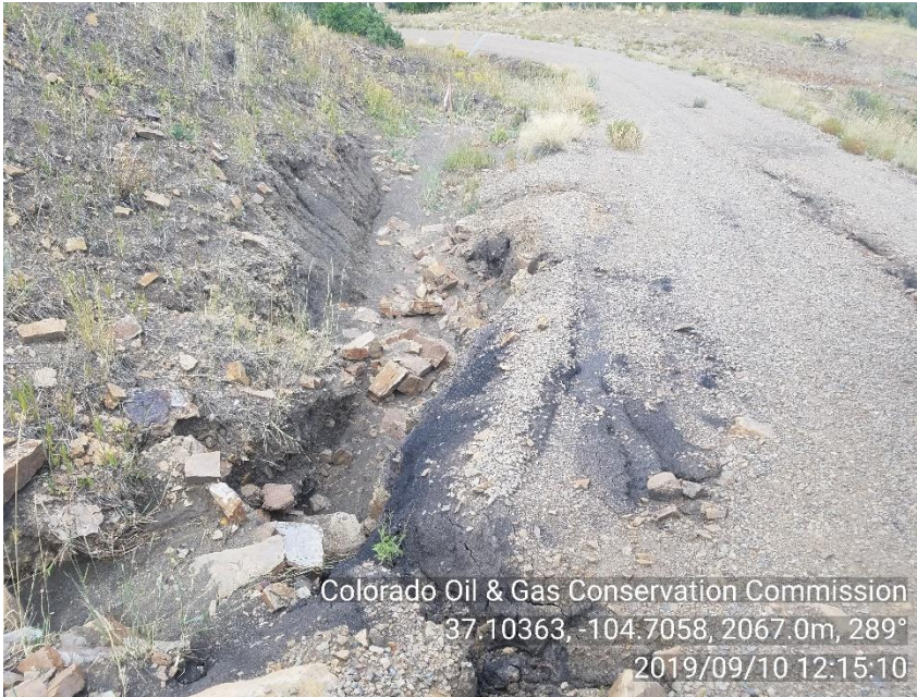
PHOTO 9: EROSION IN BMP DITCH NORTH OF LOCATION. REPAIR EROSION IN DITCH, ADD ADDITIONAL BMP'S TO SLOW STORM WATER FLOW AND PREVENT FURTHER EROSION. COMPLY WITH RULE 1002.f. CA DATE 11-10-19
