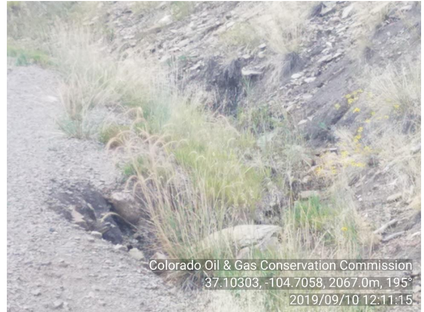
PHOTO 4: EROSION IN BMP DITCH NORTH OF LOCATION. REPAIR EROSION IN DITCH, ADD ADDITIONAL BMP'S TO SLOW STORM WATER FLOW AND PREVENT FURTHER EROSION. COMPLY WITH RULE 1002.f. CA DATE 11-10-19
