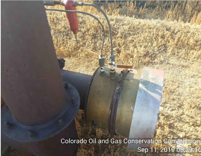
Photo 3 fuel gas to burner on separator is closed
