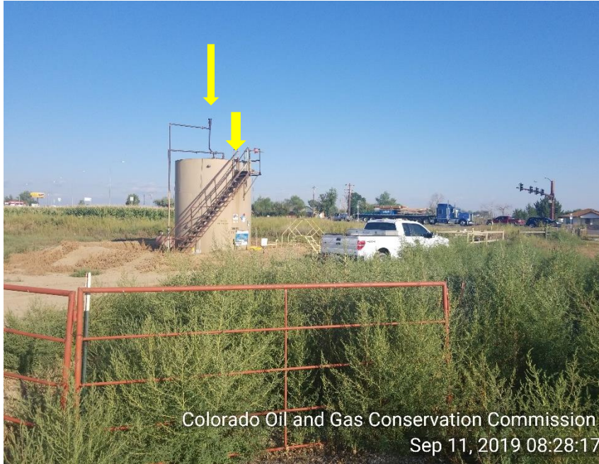
Photo 1 entrance to location. WEEDS. Gauge hatch and Pressure relief valve venting. See video
