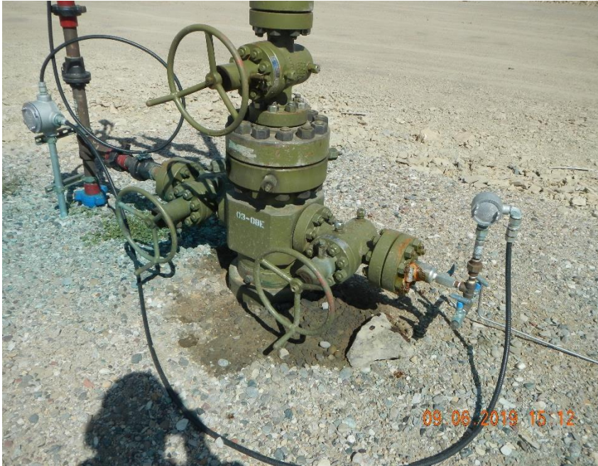
Stain soil around well heads.
