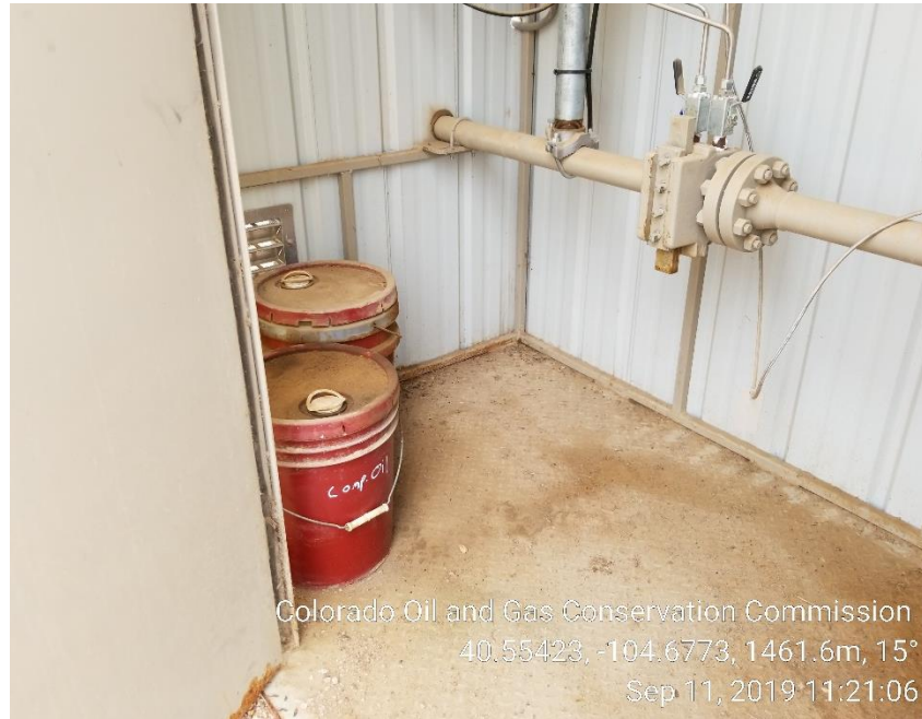
Photo 7: Storage of unknown contents in gas meter hosue.
