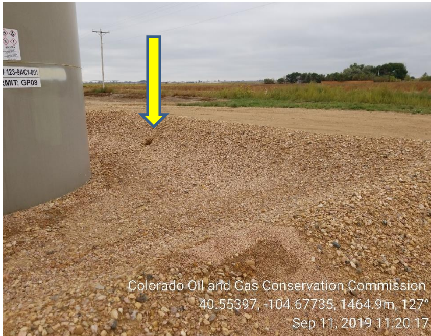
Photo 5: Hole in berm (south)
