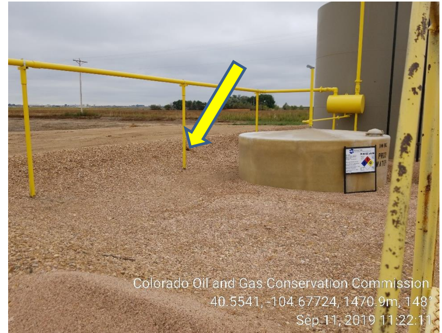
Photo 6: Hole in berm (east)
