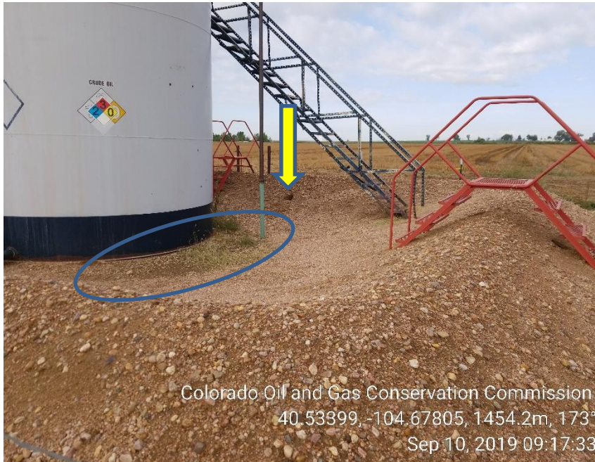
Photo 5: Weeds/Hole in berm wall
