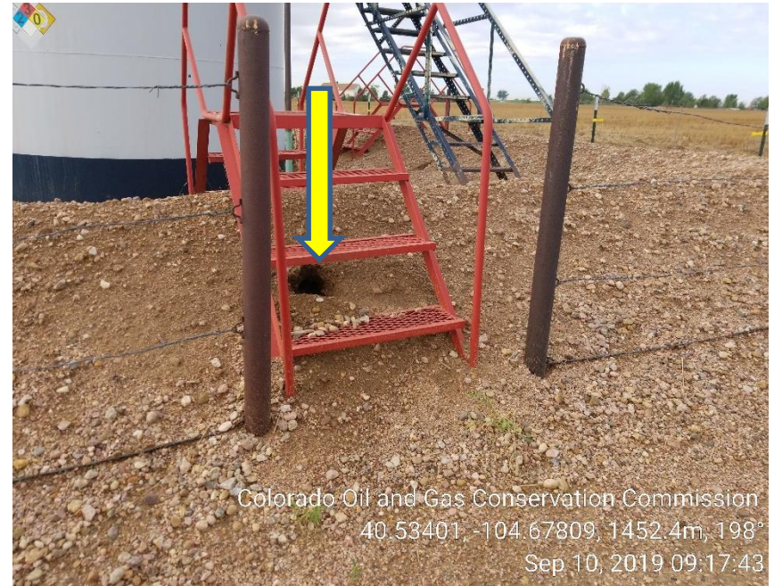
Photo 6: Hole in berm wall
