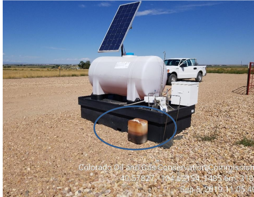
Photo 3: Container not in containment
