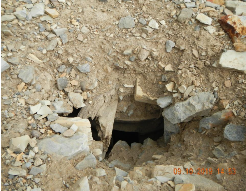
Subsidence of rathole at well EF03B.
