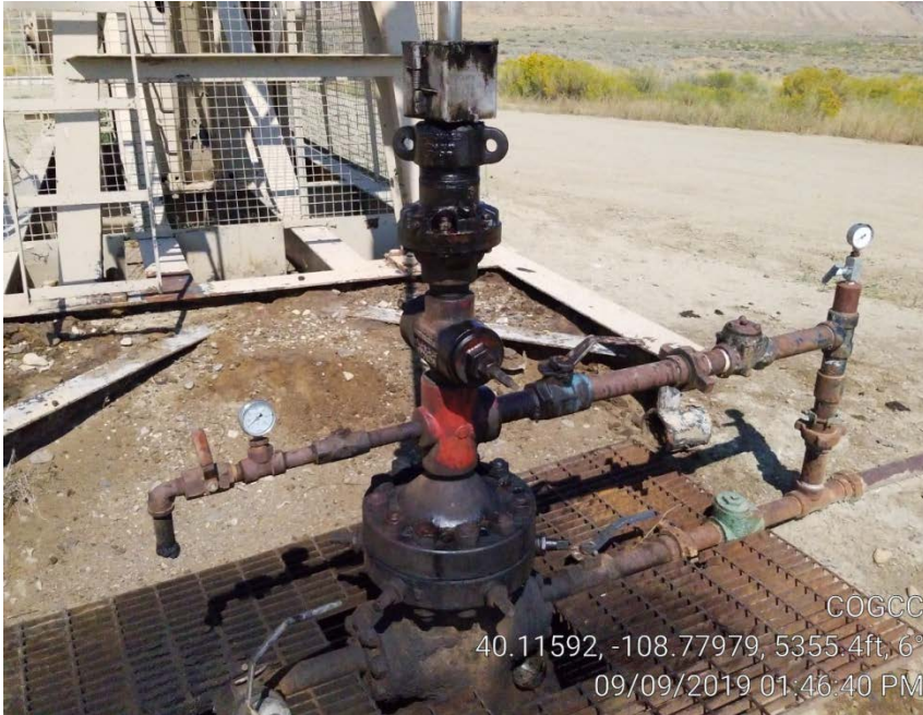
Photo 2. Well head & front of pump jack.
