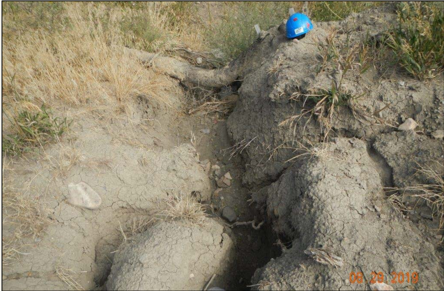
Photo 9. View of erosional channel approximately 3 feet wide and deep within the northern project area. Sediment laden stormwater flows off of the project area in this location.
