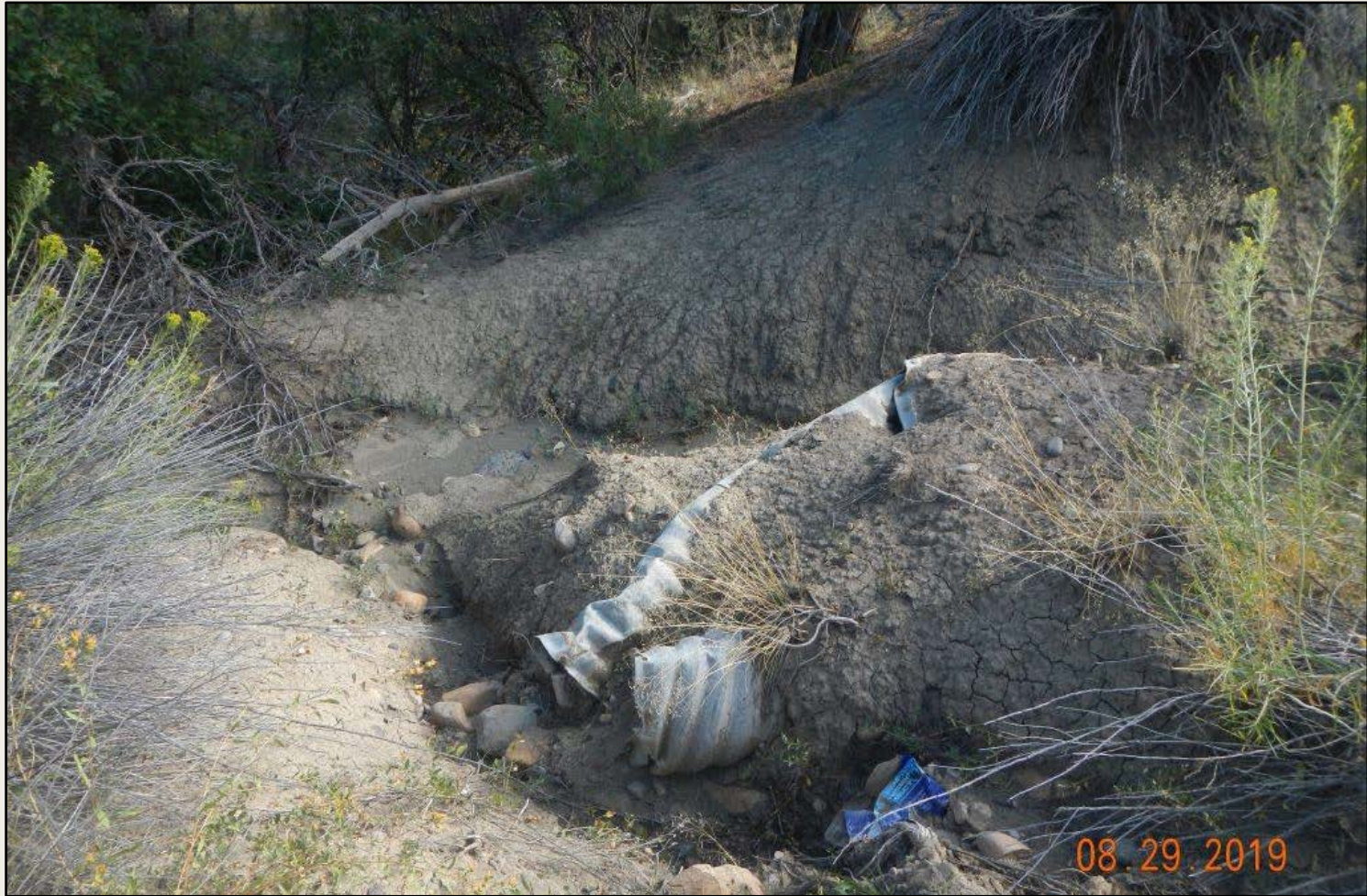
Photo 14. View of area along the access road where a blocked culvert has resulted in significant headcut erosion up to approximately 4 feet wide and deep. Culvert in photo is debris and no longer in place. Sediment laden stormwater flows off of the project area in this location as well as multiple other areas along the access road.
