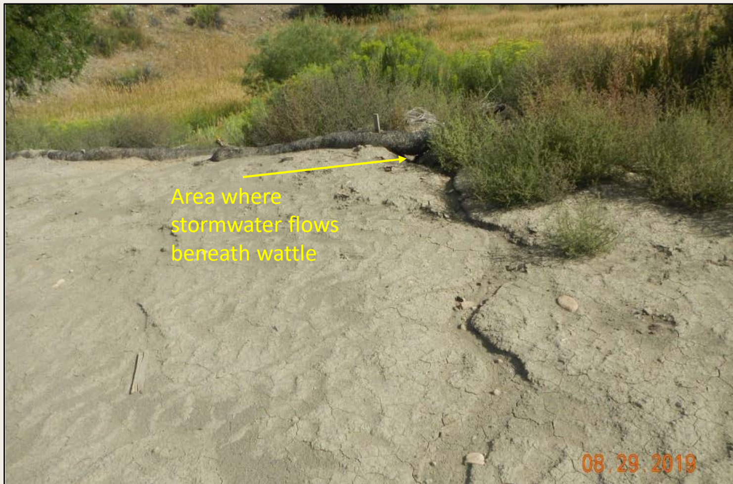
Photo 5. View of erosional channeling where concentrated stormwater and sediment flows off of the northeastern edge of the well pad. Wattles are failed, and are not adequate stormwater BMPs in this area.
