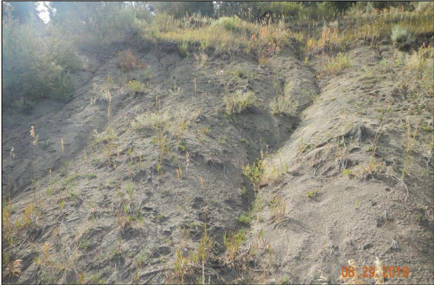
Photo 8. View of erosional rilling and bare soils on the well pad cut-slope. Evidence of erosional undercutting observed at top of slope.
