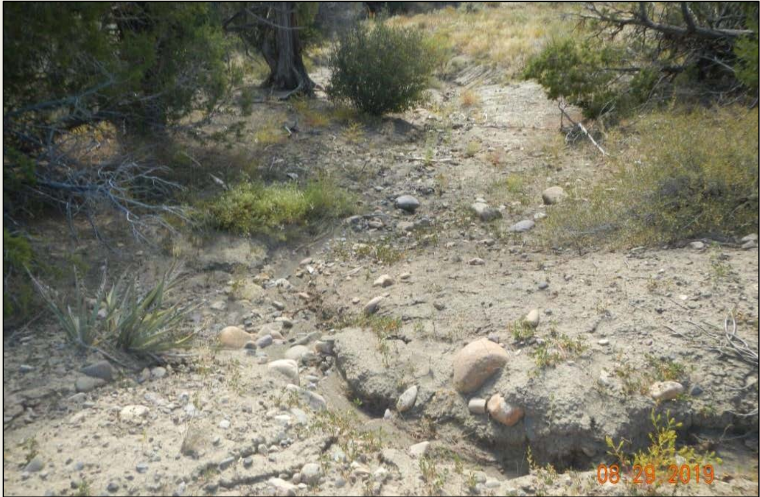
Photo 13. View of area where roadside stormwater flows are diverted without erosion or sediment controls, and erosion is occurring within a channel that is approximately 1 foot wide and deep, scouring and channeling continues downstream.
