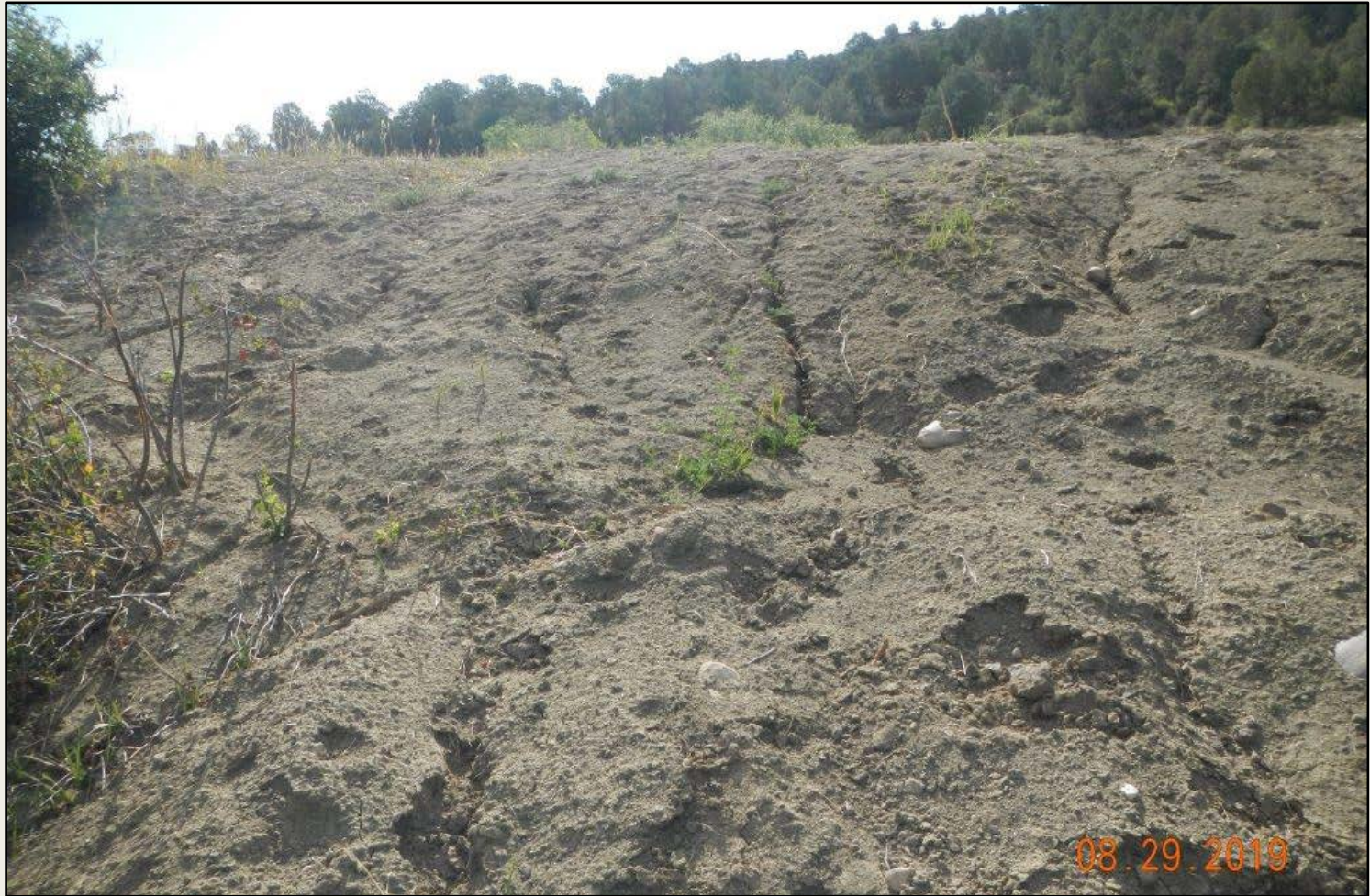
Photo 4. View of disturbed soils northwest of well pad and along flowline with bare soils on slope that are eroding.
