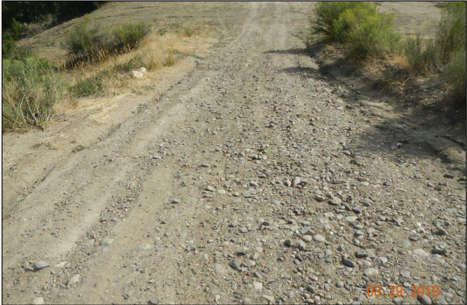
Photo 9. View of current and developing erosional channeling along the access road near the well pad entrance.
