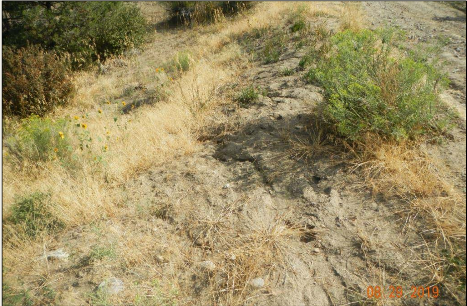
Photo 8. View of erosional channeling along the access road near the well pad entrance, facing down-slope.
