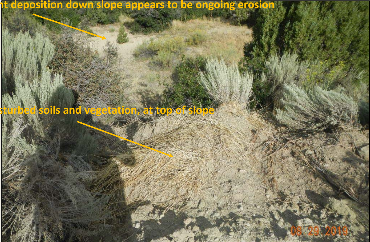
Photo 5. View of area in the western project area that is disturbed, and evidence of ongoing erosion on fill slope as well as sedimentation observed.
