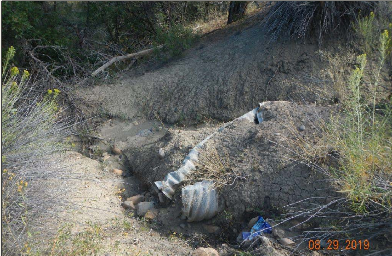
Photo 14. View of area along the access road where a blocked culvert has resulted in significant headcut erosion up to approximately 4 feet wide and deep. Culvert in photo is debris and no longer in place.
