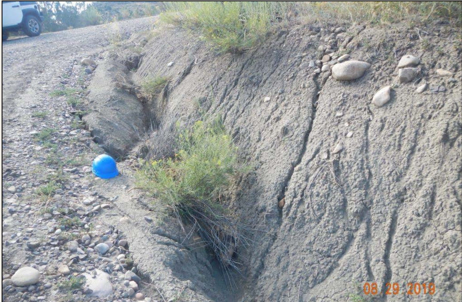
Photo 11. View of erosional channeling and rilling along the edge of the access road.
