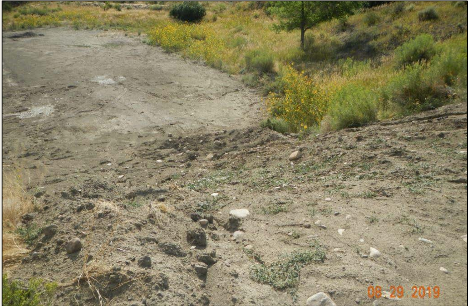
Photo 10. View of disturbed soils, unprotected within the northeastern project area, facing downslope. Rilling observed.
