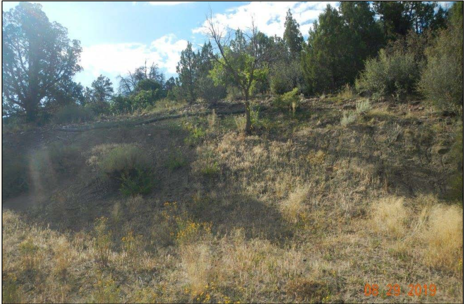
Photo 2. View of southern cut-slope, largely comprised of annual weeds such as cheatgrass ( Bromus tectorum ) and alyssum ( Allysum simplex ) This slope is not stabilized as annual weeds, bare soils, and rilling observed.
