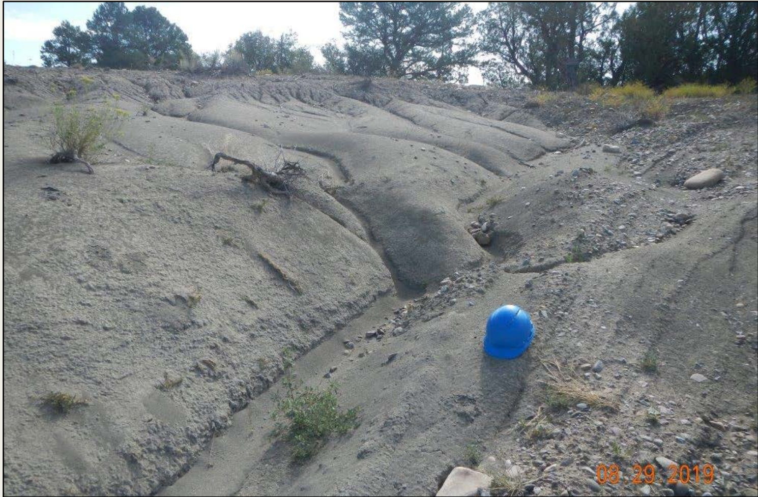
Photo 12. View of area of significant erosional channeling, scouring, and destabilized cut-slope along the access road.
