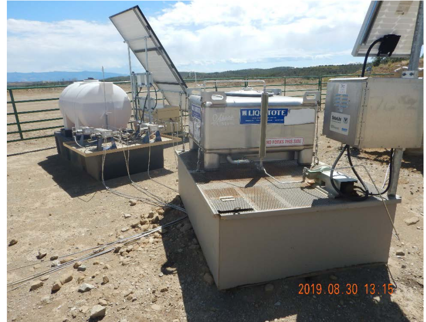
Photo #4 – Chemical storage tank and process pipe pump controls located inside fenced wellhead area.
