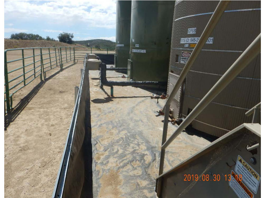
Photo #6 – View into east side of tank battery secondary containment.
