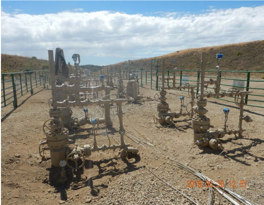
Photo #9 – Overview of wellhead area from north. No audible gas leaks were detected in this area on inspection date.
