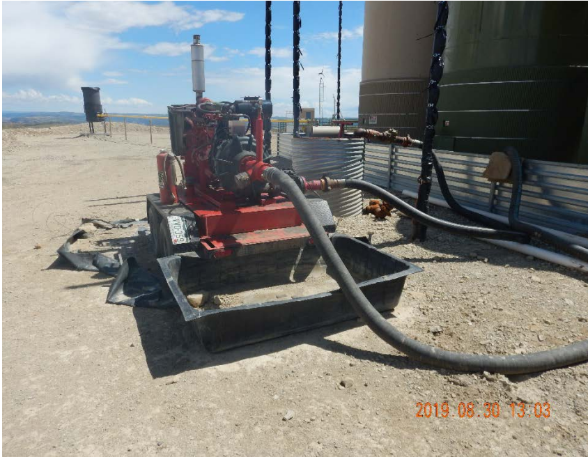
Photo #5 – Trailer pump with secondary containment on north side of tank battery.
