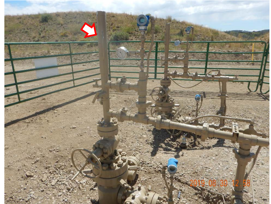
Photo #10 – 596-31A-27 wellhead. Audible rattling was observed coming from plunger lift on inspection date.
