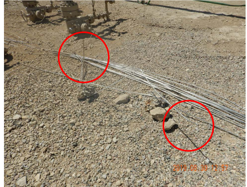
Photo #8 – Uncapped, unmarked process piping observed north of wellheads.
