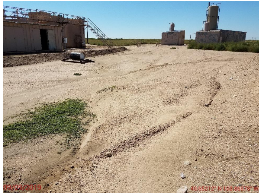
Photo 8: Photo taken from the east central area of the location, facing southwest. Photo shows stormwater erosion degradation on location.
