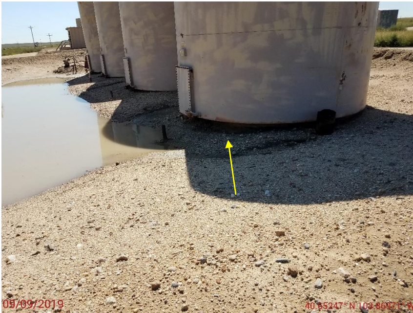
Photo 13: Photo taken from the tanks on the north end of the location. Photo shows stormwater erosion appears to be undermining the tanks.
