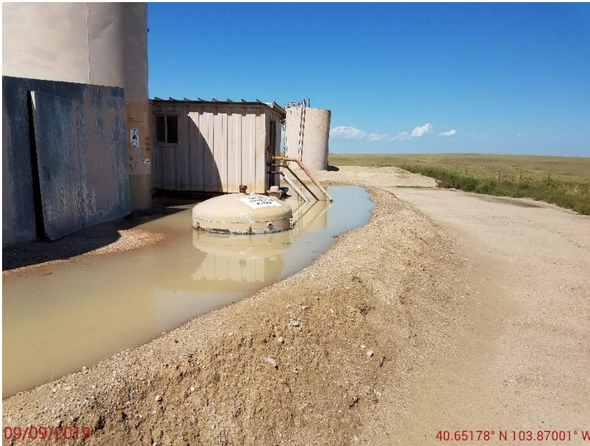
Photo 5: Photo taken from the east end of the tanks on the southeast end of the location. Photo shows secondary containment does not appear to be sufficient to contain the contents of the largest single tank and sufficient freeboard to contain precipitation.
