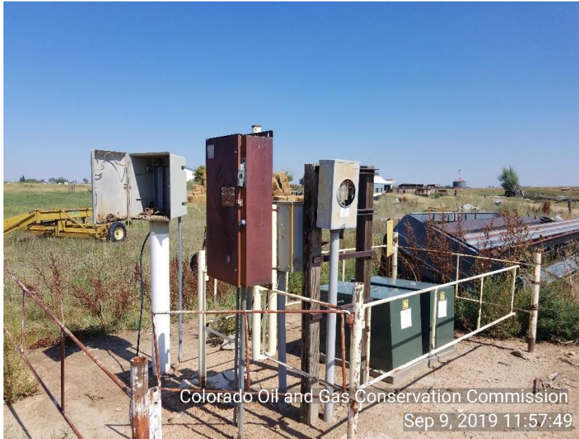
Photo 11 Unused equipment: Electric panel Meter has been pulled.
