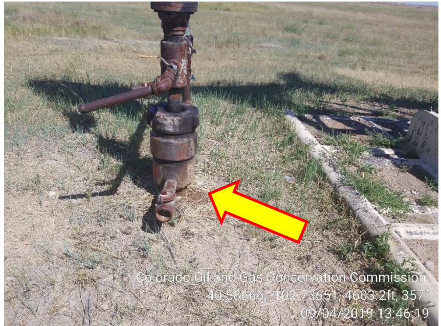
Photo 4 – Stained Soil at Wellhead
