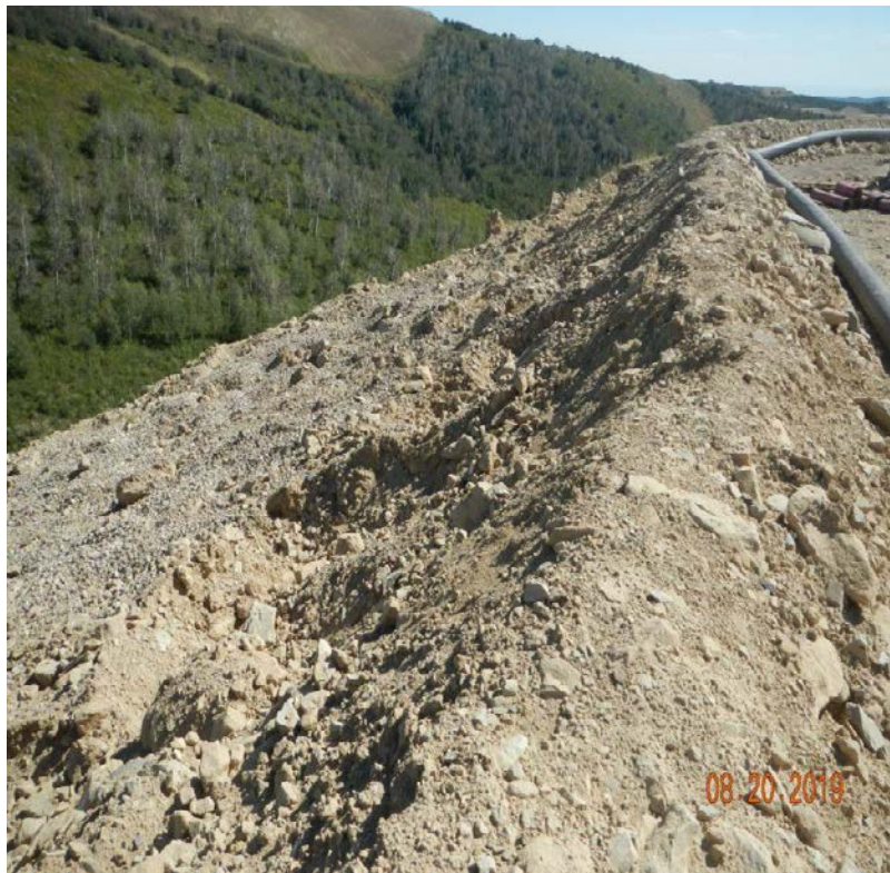
Photo#2: Fill slopes remain unstable.
