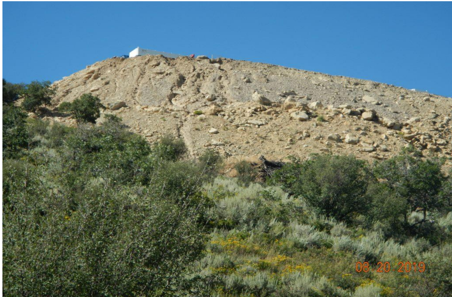
Photo#6: Fill slopes remain unstable and erosion is occurring.
