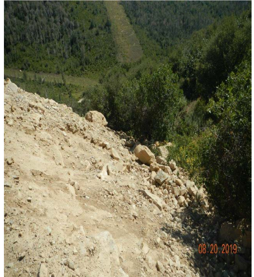
Photo#5: Fill slopes remain unstable.
