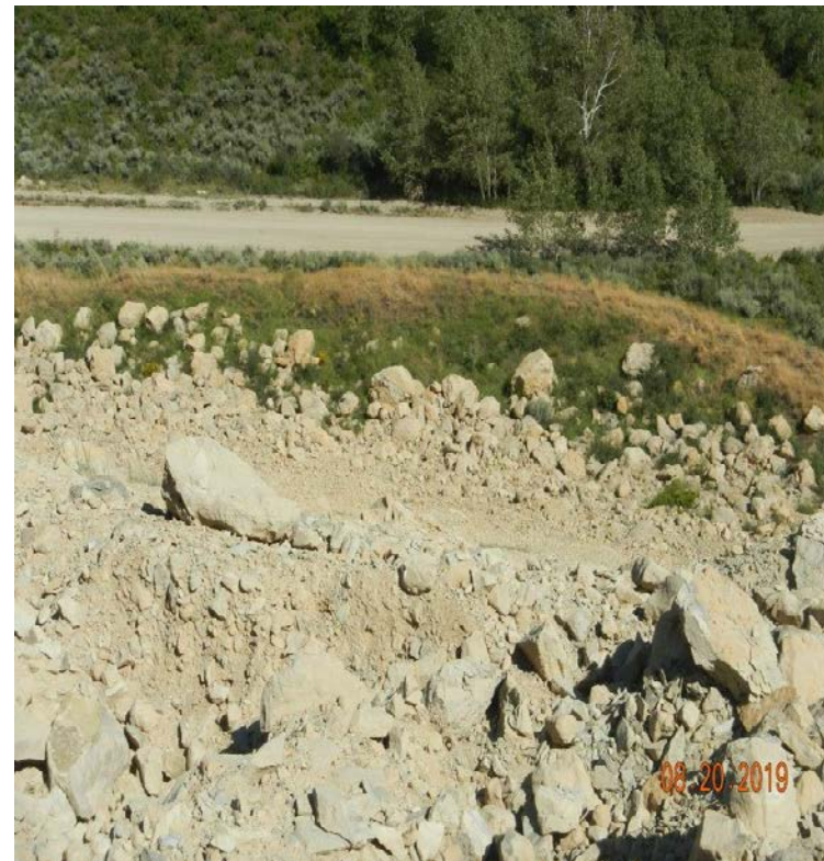
Photo#3: Fill slopes remain unstable.
