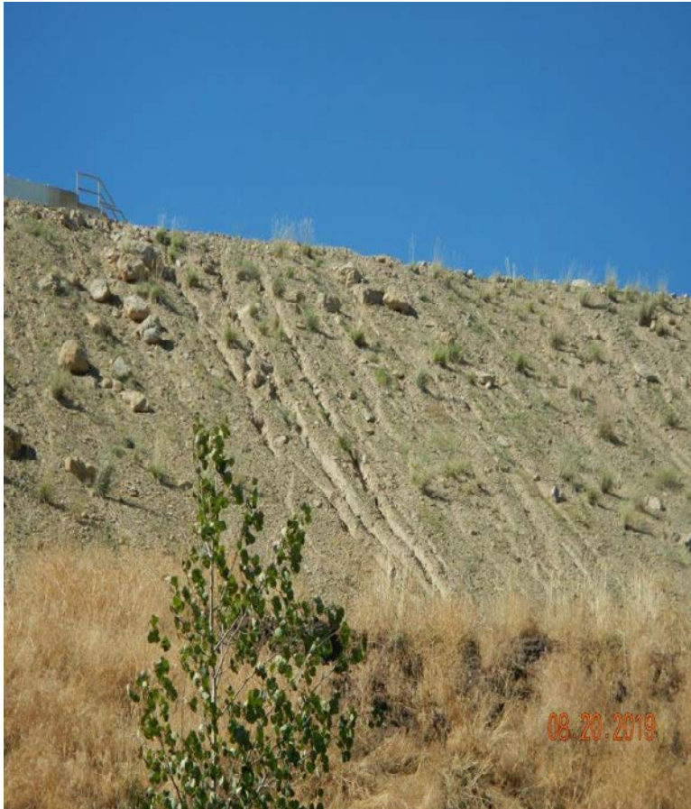
Photo#7: Fill slopes remain unstable and erosion is occurring.
