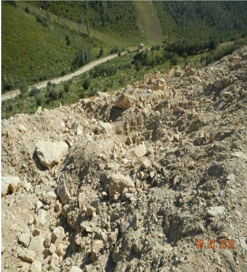
Photo#4: Fill slopes remain unstable.
