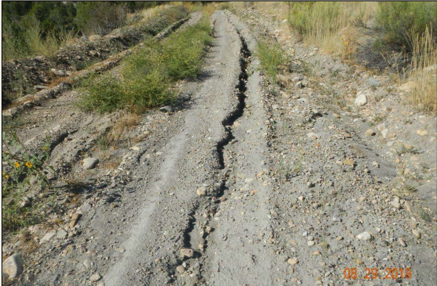
Photo 7. View of erosional channeling and sedimentation on the access road.
