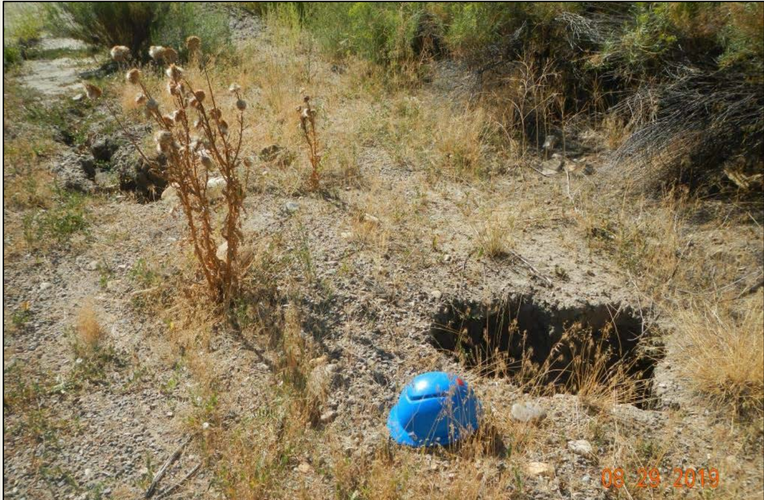
Photo 5. View of erosional tunnels within the northwestern fill slope, near the well pad entrance.
