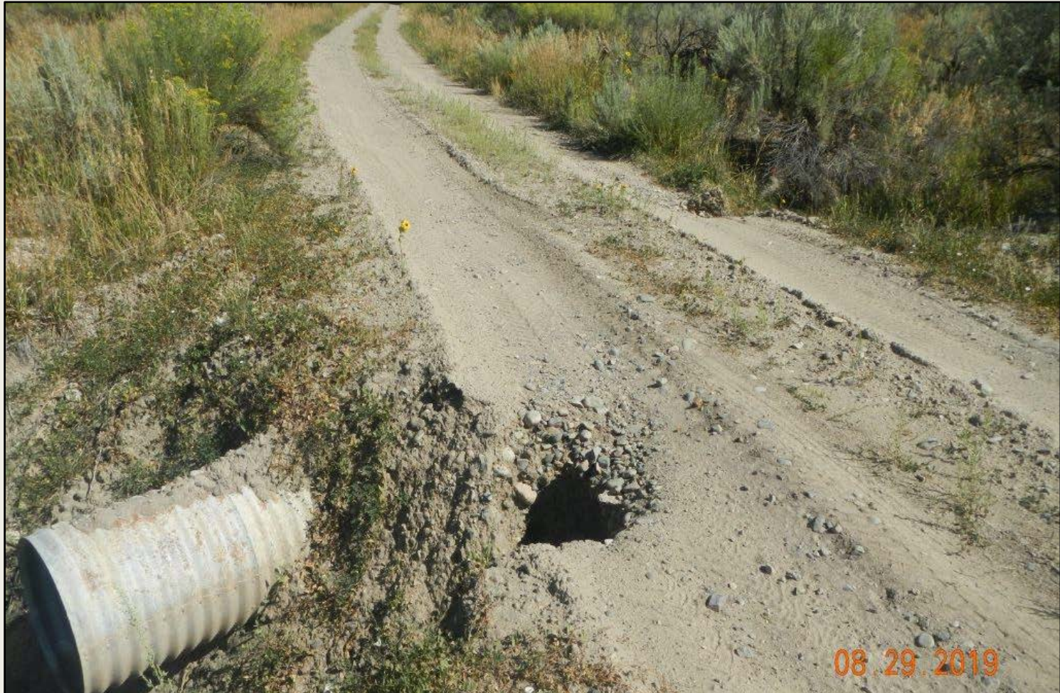
Photo 8. View of erosional downcutting along both sides of culvert along access road. This is compromising the integrity of the access road and needs to be repaired.
