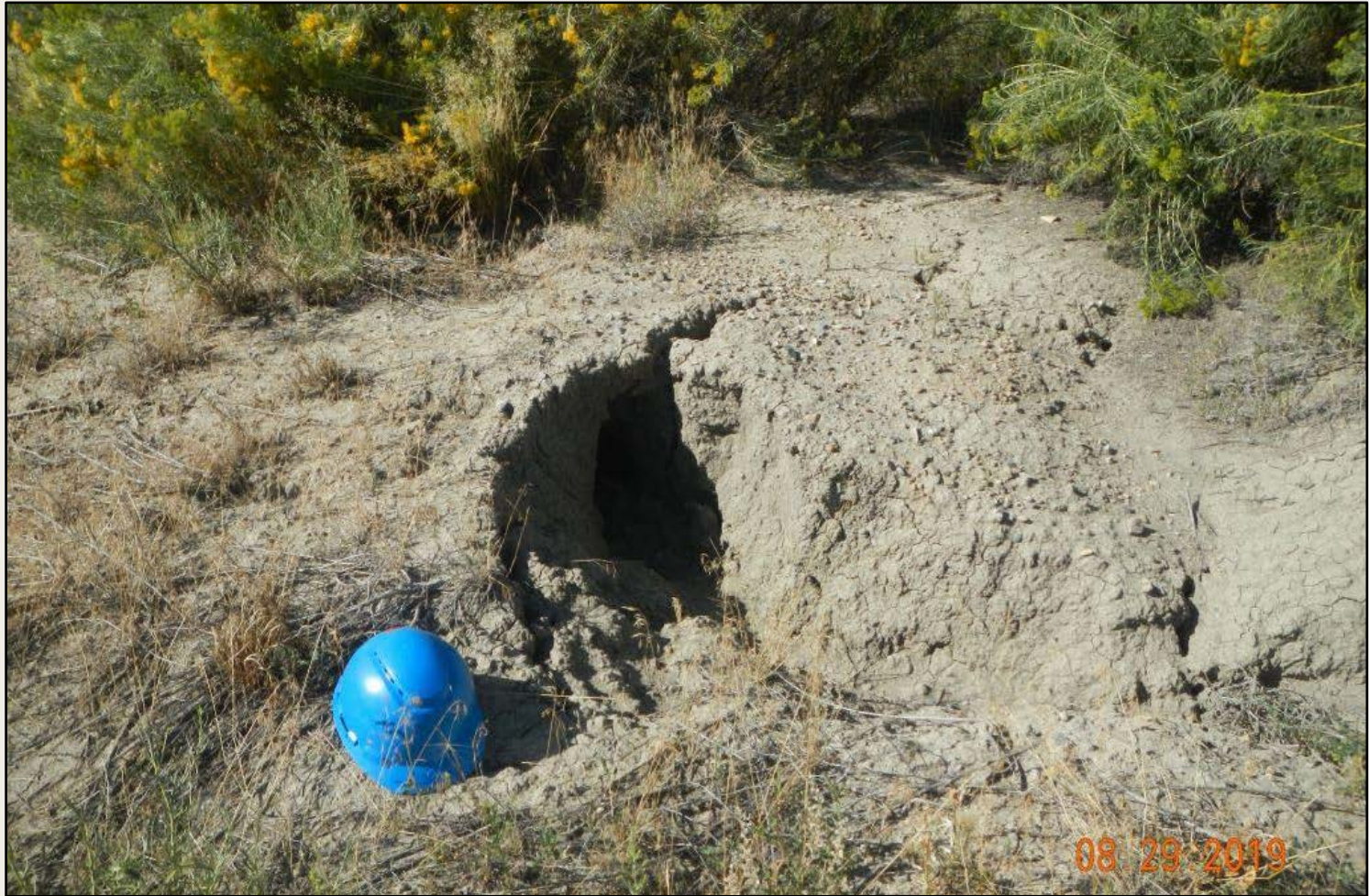
Photo 4. View of erosional tunnel within the southeastern fill slope.
