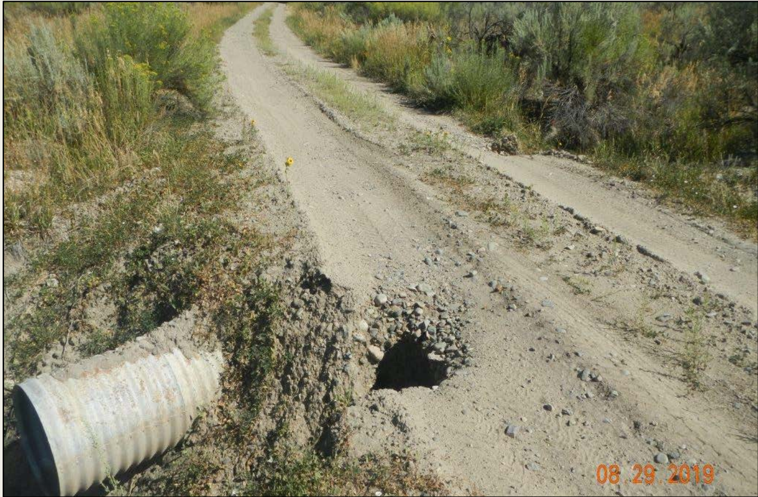
Photo 5. View of erosional downcutting along both sides of culvert along shared access road. This is compromising the integrity of the access road and needs to be repaired.
