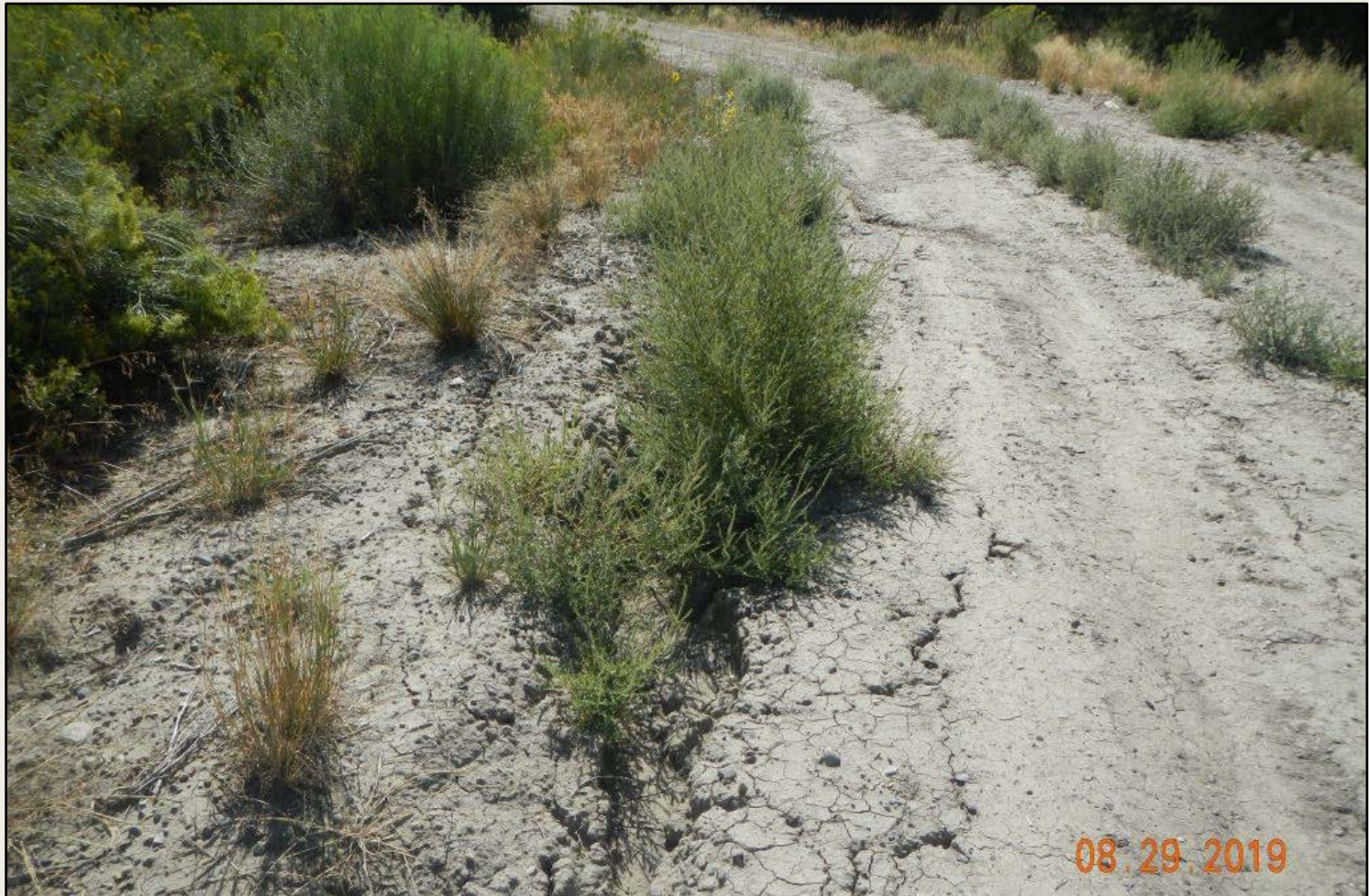
Photo 3. View of erosional channeling at the well pad entrance facing eastward.
