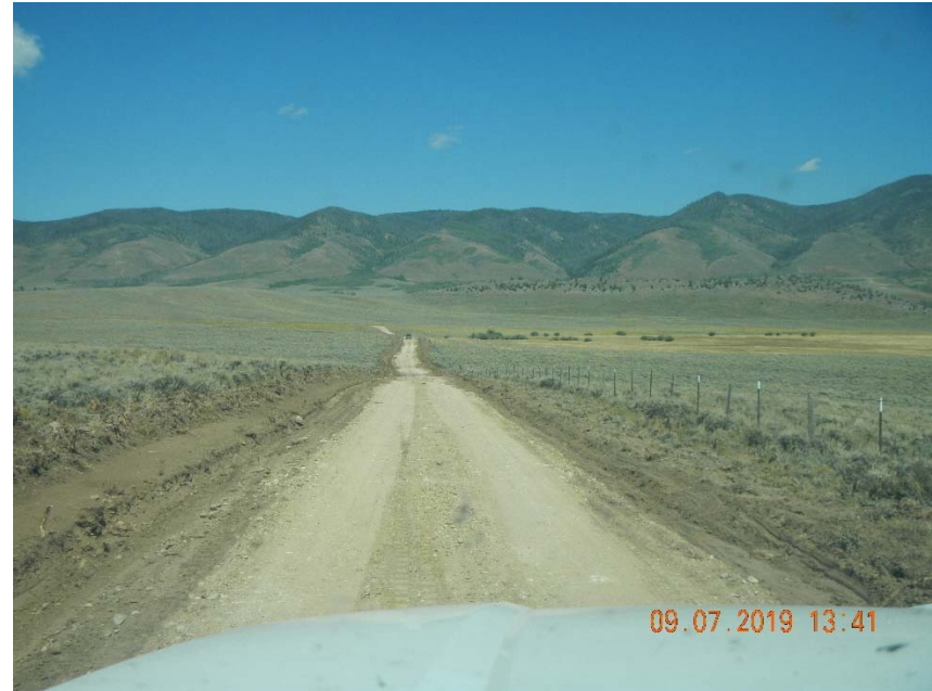
Photo 6. Gravel added to access road, no stormwater controls on perimeter of road.
