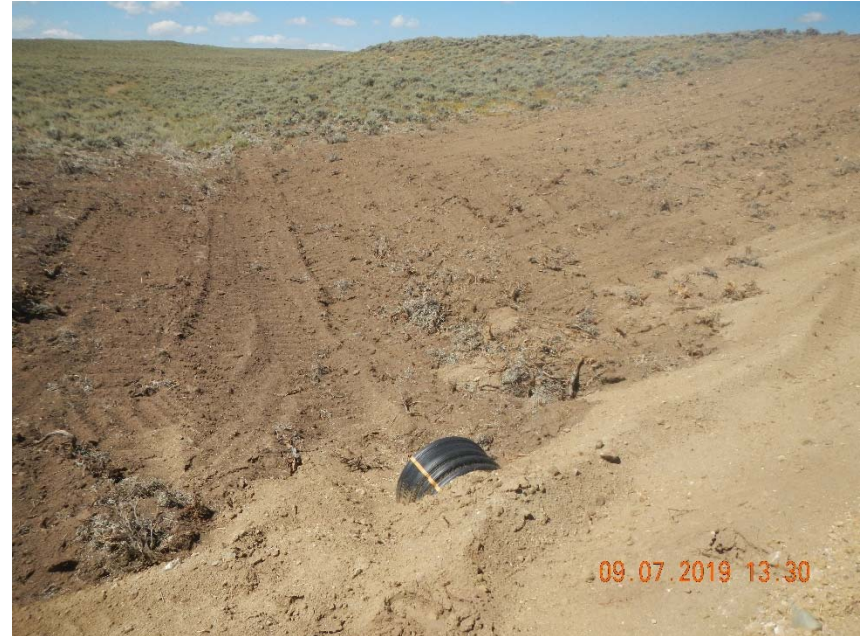
Photo 10. No stormwater controls observed on west, uphill, side of drainage crossing.
