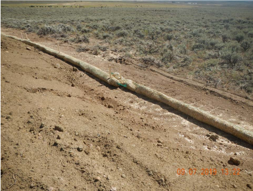
Photo 7. Wattles installed on some of location perimeter. Wattles not trenched.
