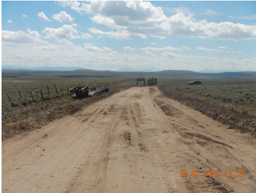
Photo 5. Surface disturbance increase, trucks driving/parking on side of access road. Gravel added to access road, no stormwater controls on perimeter of road.
