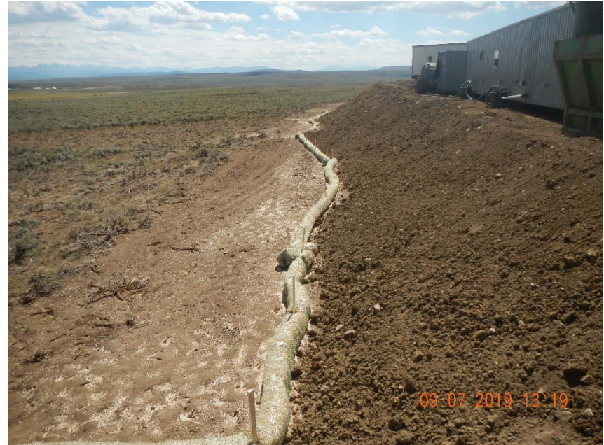
Photo 8. Wattles installed on some of location perimeter. Wattles not trenched.
