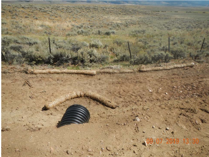
Photo 9. Wattles installed on east side of drainage crossing. Wattles not trenched. No other controls observed.
