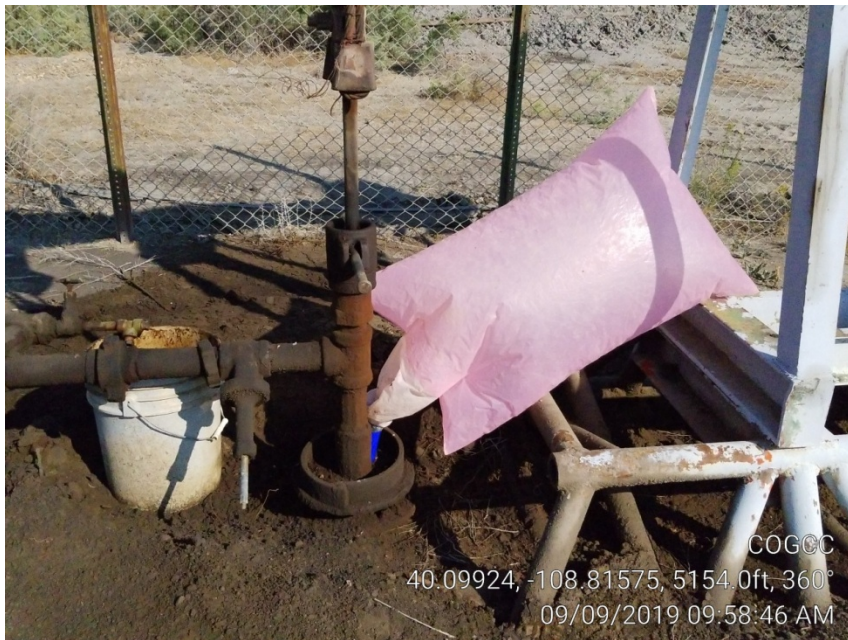
Photo 7. Gas vented into 3 cubic foot bag.
