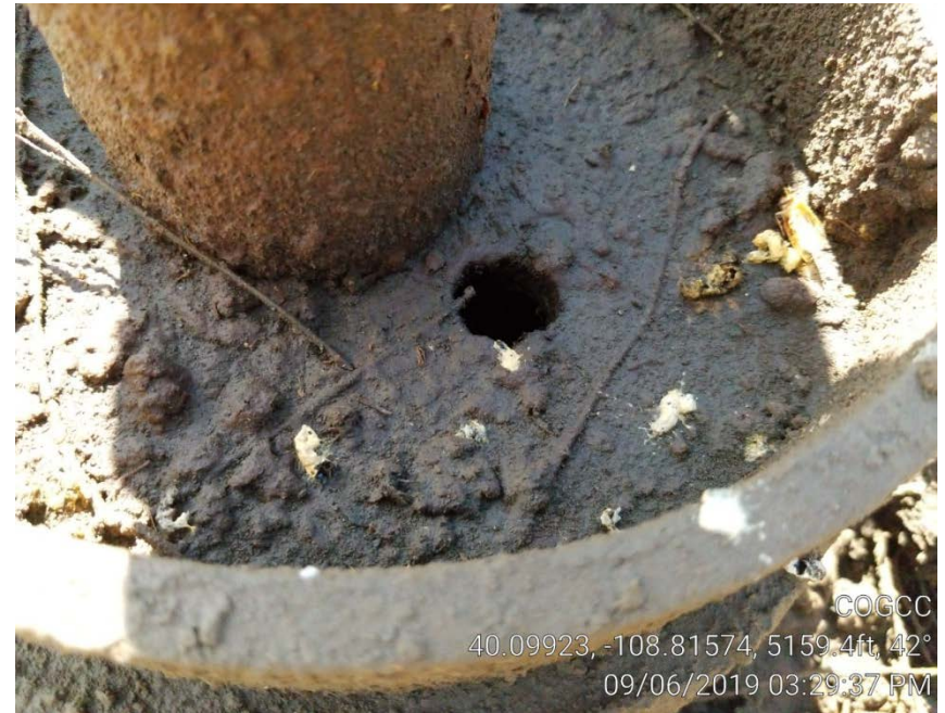
Photo 4. Casing open to atmosphere.
