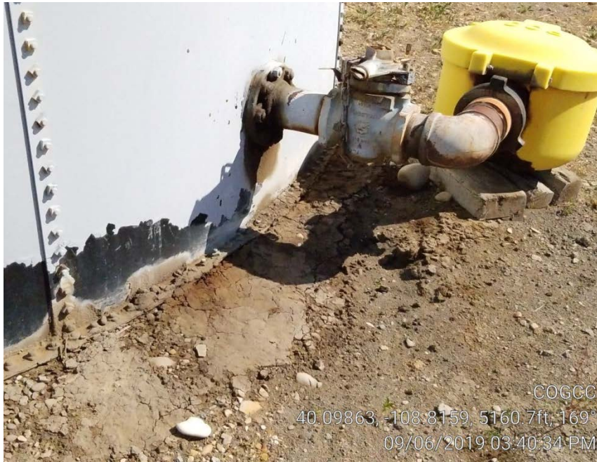
Photo 12. Stained soil next to tank.
