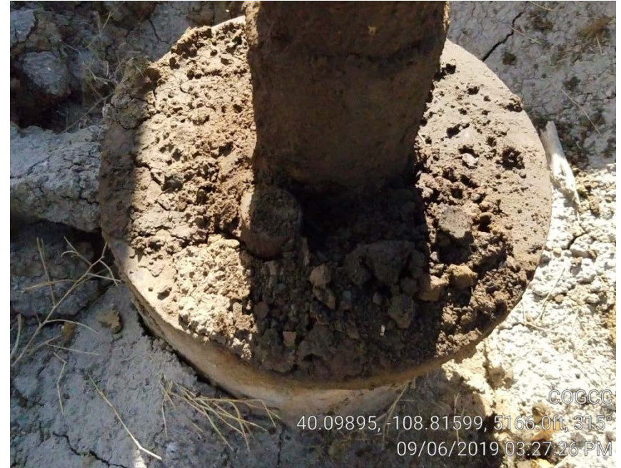
Photo 9. Casing open to atmosphere (dirt on opening) – Stagner 6.
