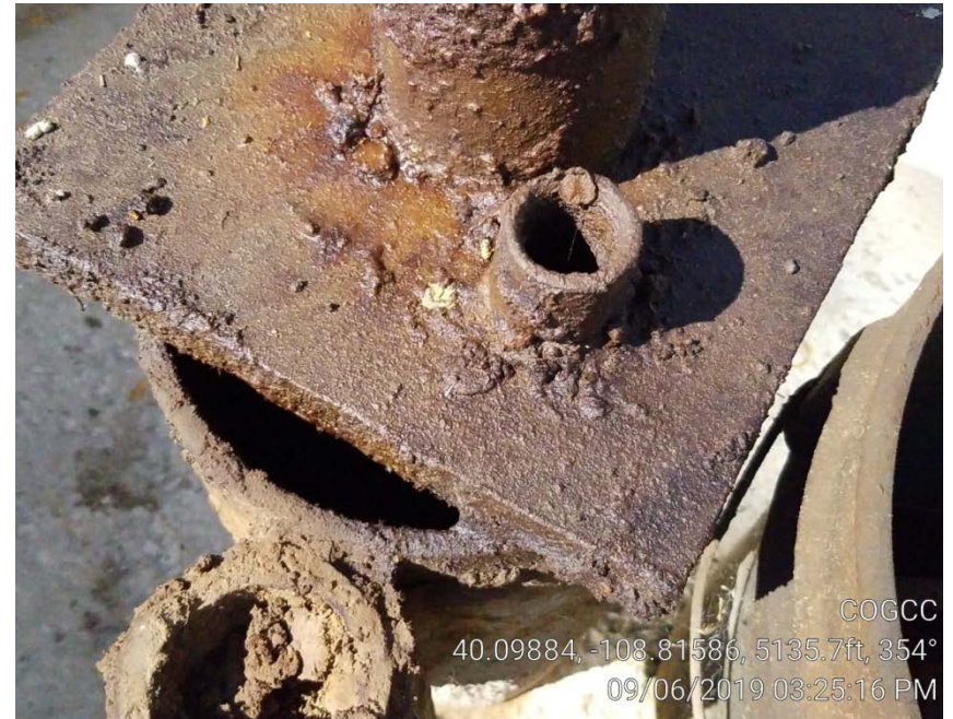
Photo 5. Casing open to atmosphere – Stagner 2.
