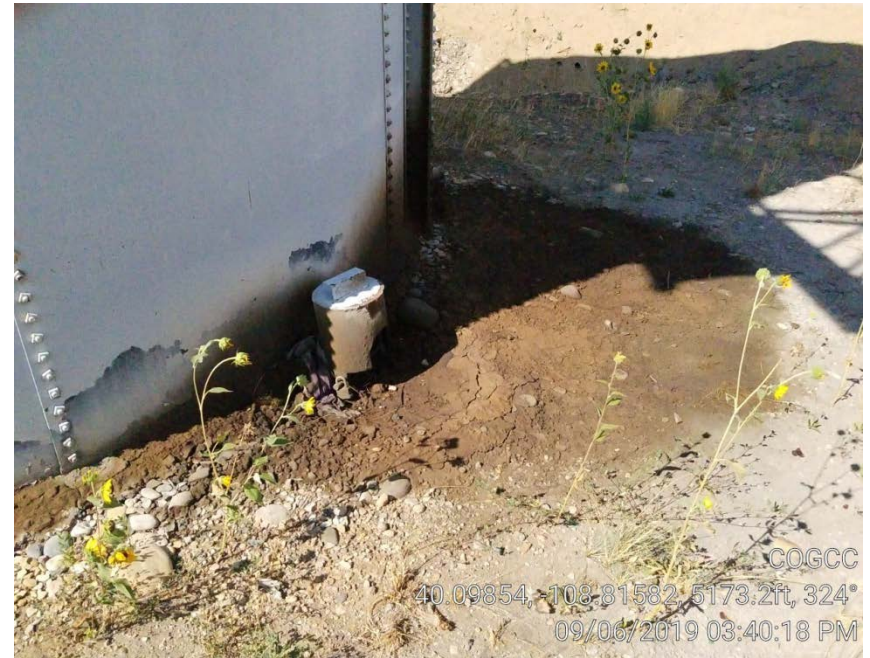
Photo 11. Stained soil next to tank.
