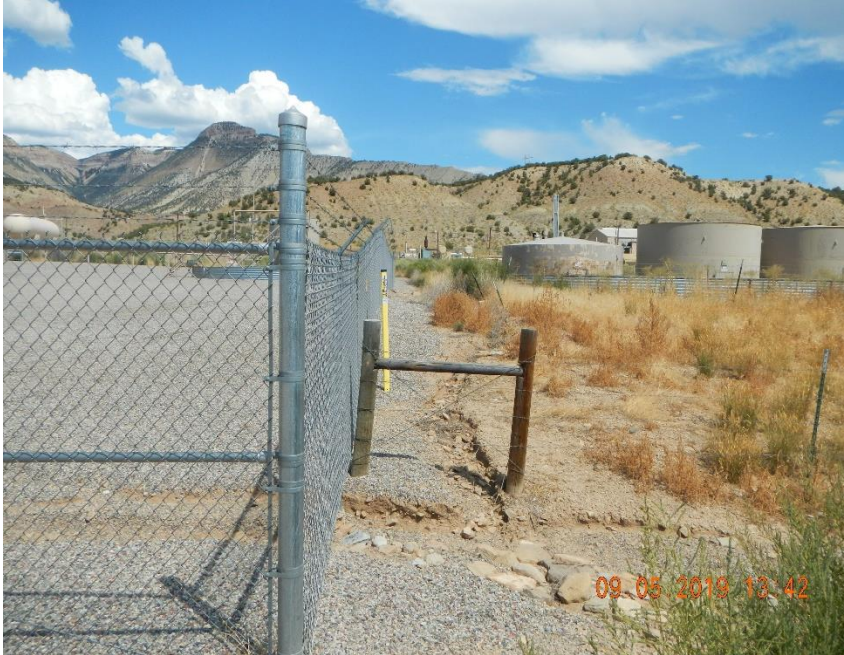
South west fence line run off ditch washing.
