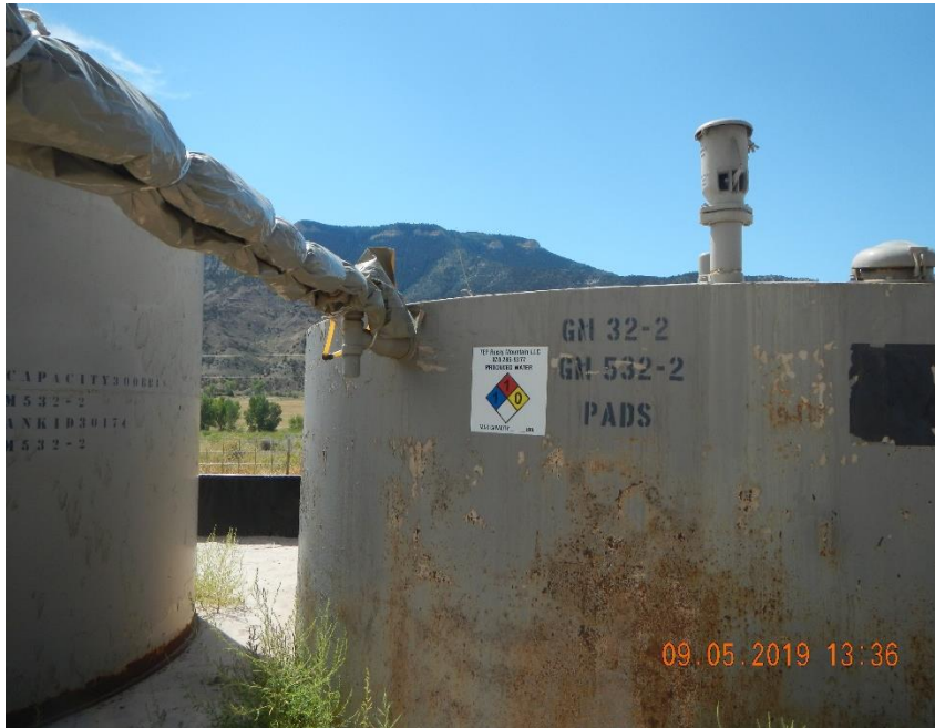
No capacity on tank label. Weeds in berm.
