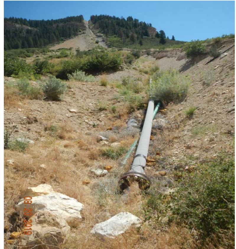
Photo#4: Flowline/pipeline from top of plateau to Location has not had trench properly filled in, stabilized or re-vegetated
