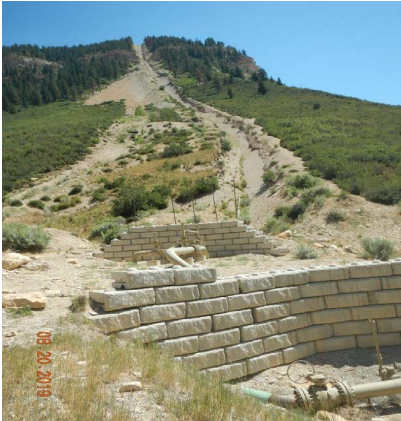
Photo#3: Flowline/pipeline from top of plateau to Location has not had trench properly filled in, stabilized or re-vegetated
