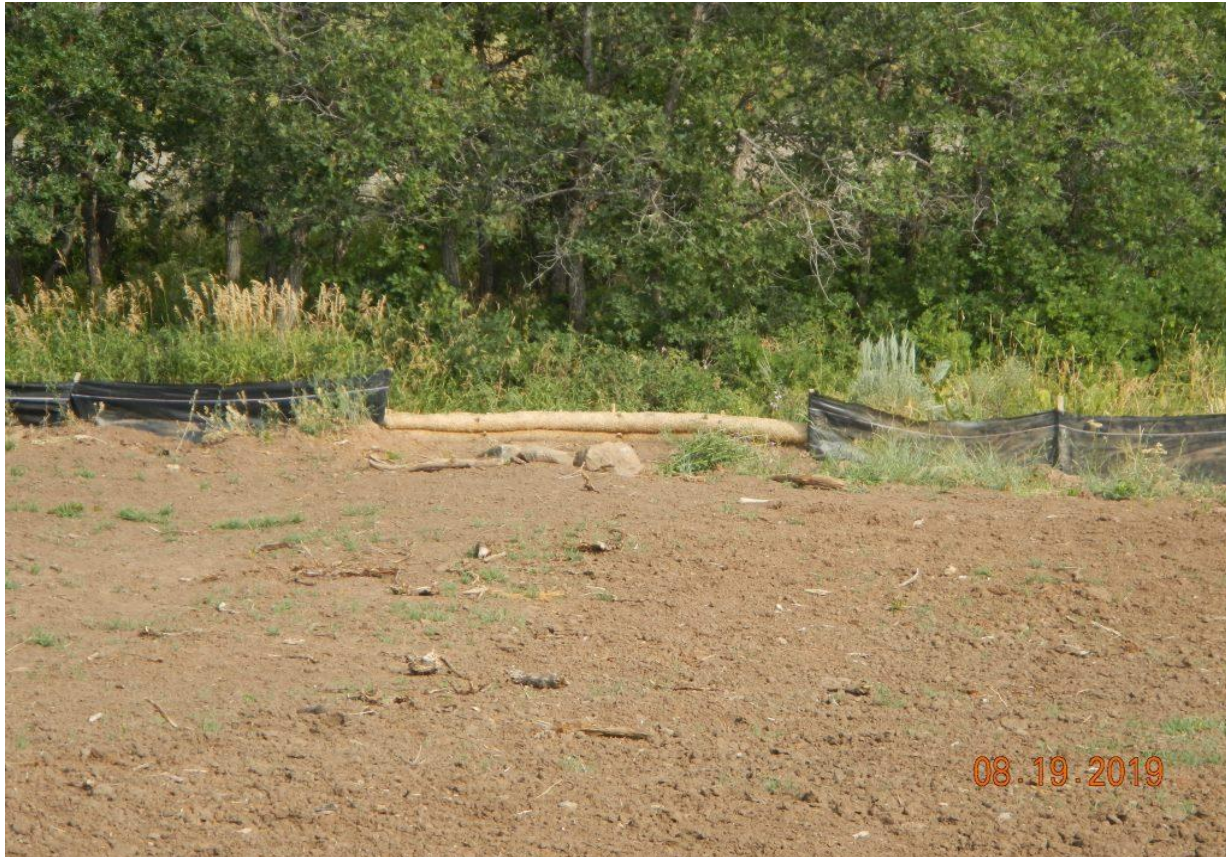
Photo#3: Stacked wattle; wattles are designed for low surface flows .
