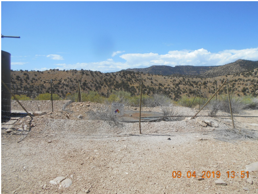
Blowdown tank with fencing and sign
