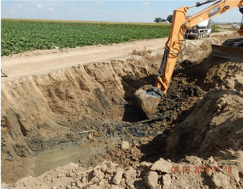
Excavation at release point; flowline being exposed. Impacted soils observed.
