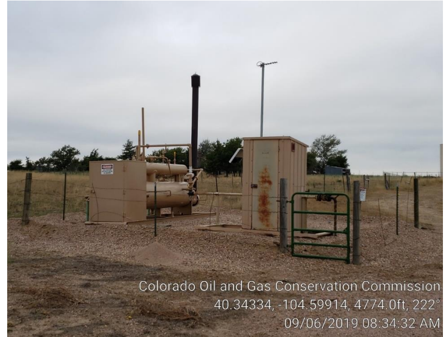
Photo #4 Separator & Meter Run
