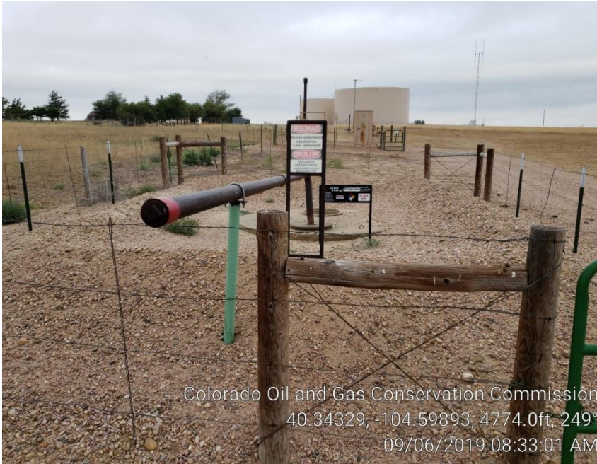
Photo #3 Produced water pit/vault
