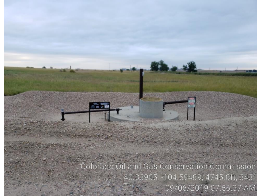
Photo # 4 Produced water vault/pit
