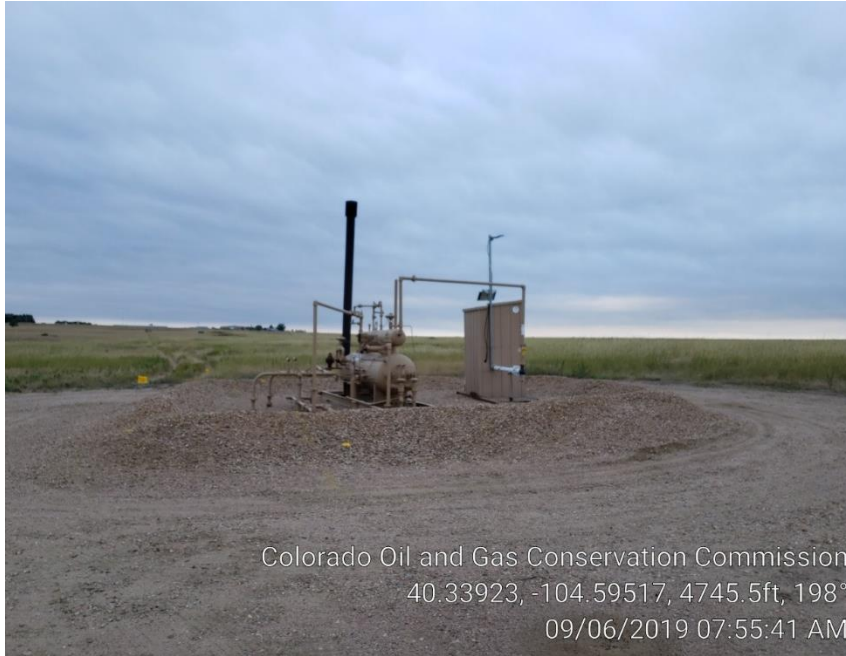
Photo # 3 Separator & Meter Run
