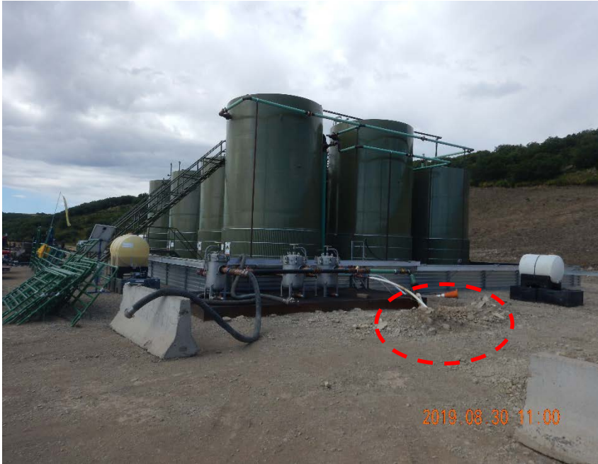
Photo #3 – Filter pots and day tanks located north and east of tank battery. Red circle denotes open excavation area.
