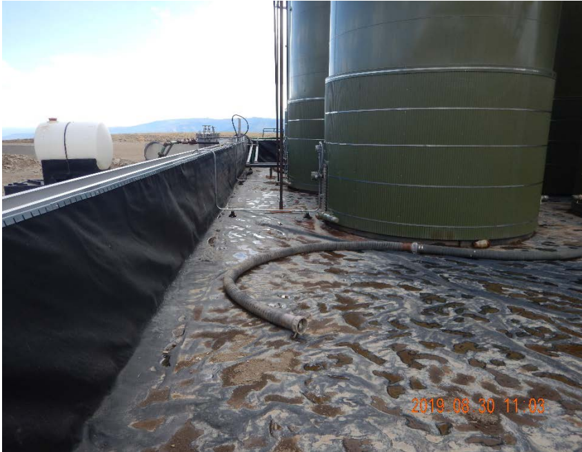
Photo #9 – Hose stored on west side of tank battery had metal fittings in direct contact with liner on inspection date. Note de minimis accumulations of fluids and soil inside of tank battery.
