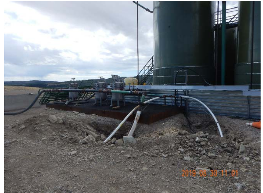
Photo #4 – Open excavations north of tank battery.
