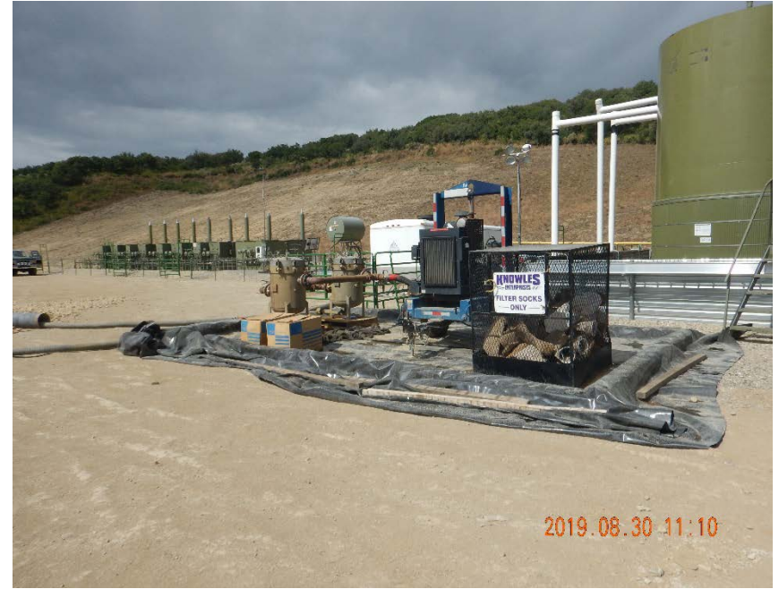
Photo #12 – Trailer pump, filter socks, and filter stock storage container on top of lined secondary containment located southeast of tank battery.
