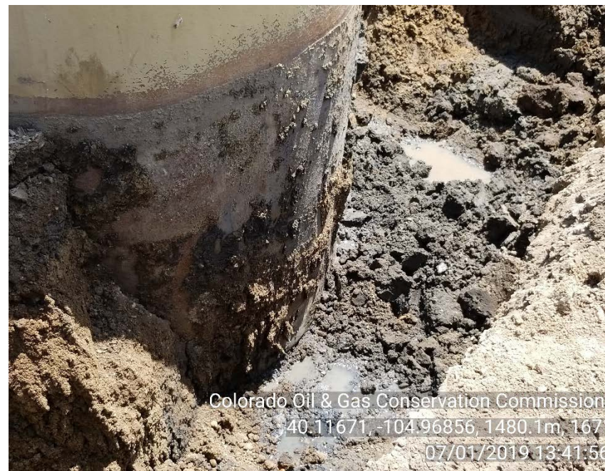
Impacted soils and ground water observed in the excavation.
