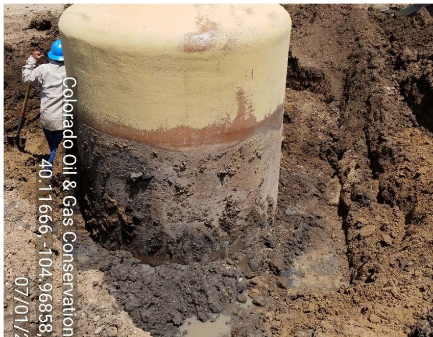
Partially buried produced water vessel in open excavation.
