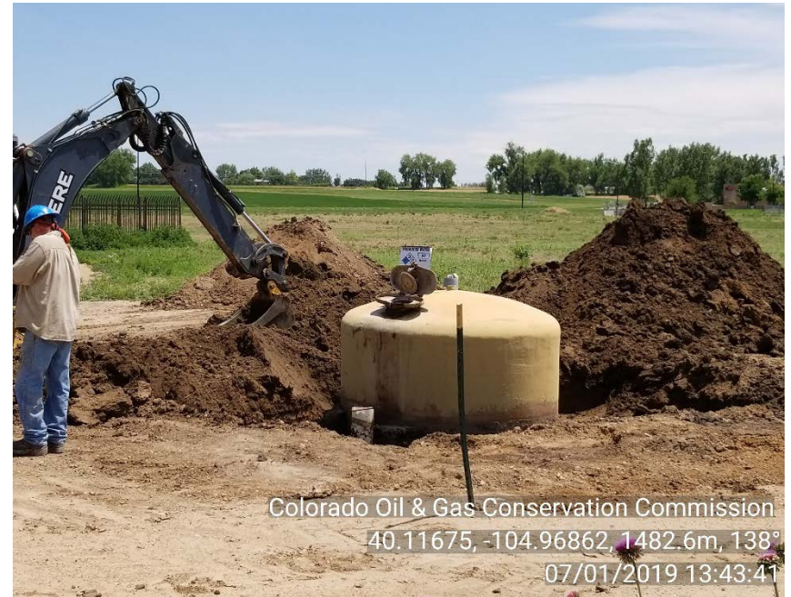
Partially buried produced water vessel being removed.
