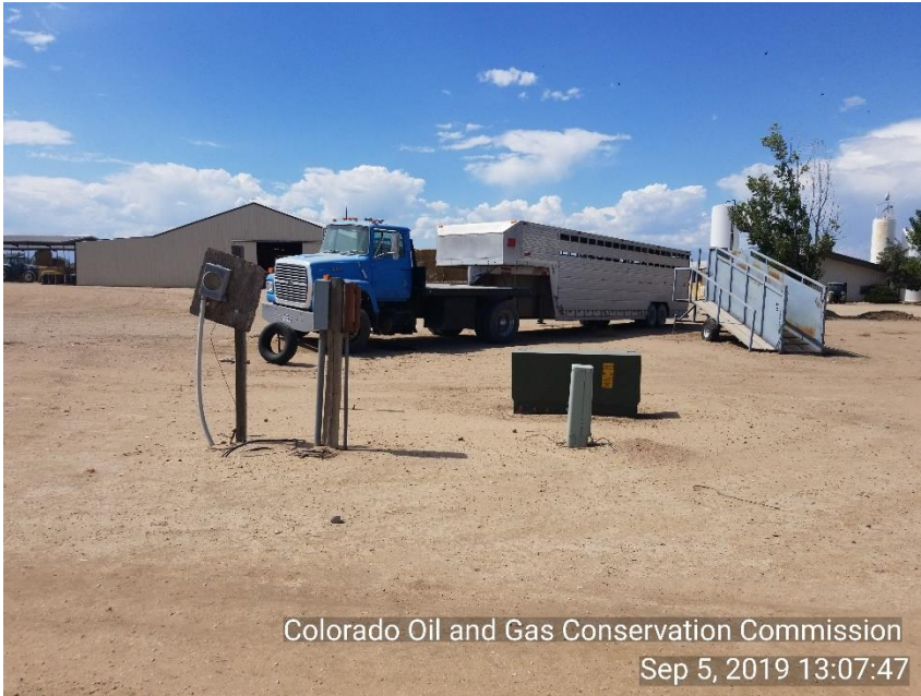
Photo 5 Unused equipment: Electric panel meter has been pulled.
