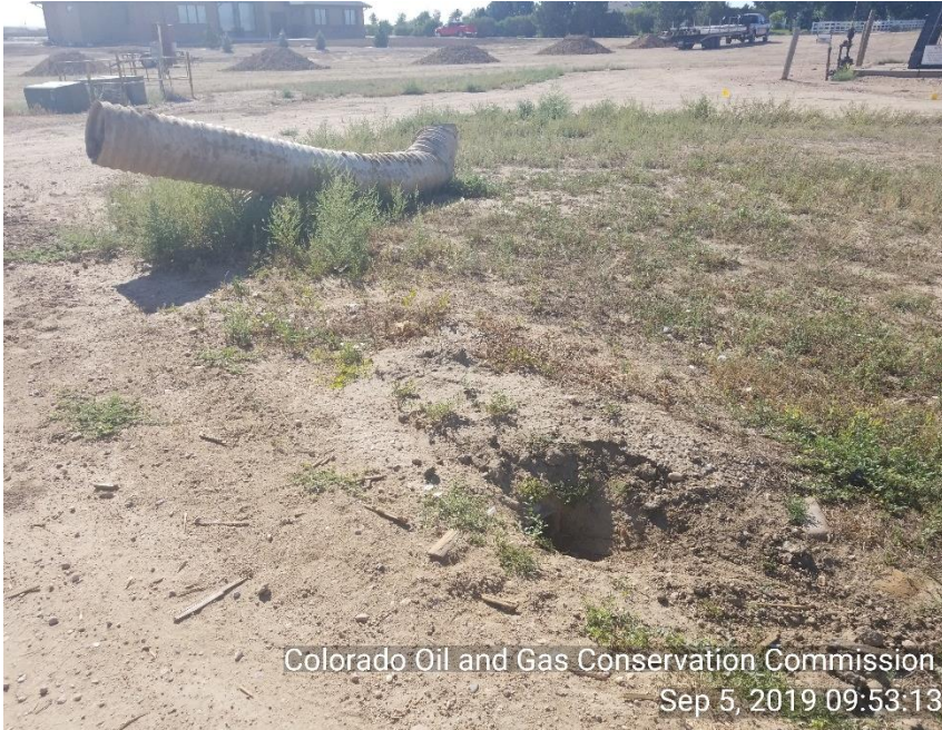
Photo 1 Culvert to access road to location inlet appears to be plugged and ditch not maintained to culvert. Part of culvert has been removed.
