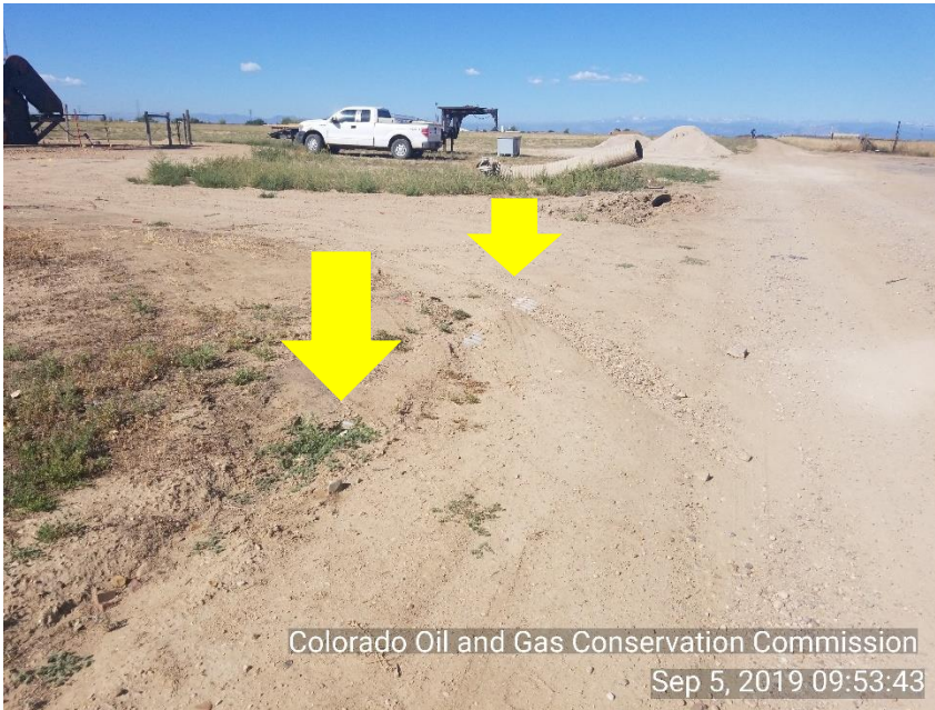
Photo 3 Culvert to access road to location outlet is plugged and exposed culvert not properly covered.
