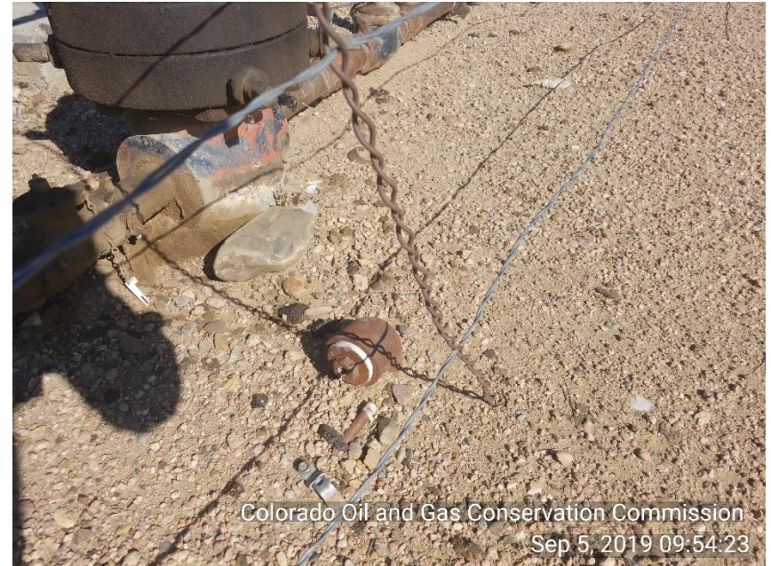
Photo 4 What appears to be the Braden head piping Mechanical issue: 1/4 inch line has been removed and is laying on ground.
