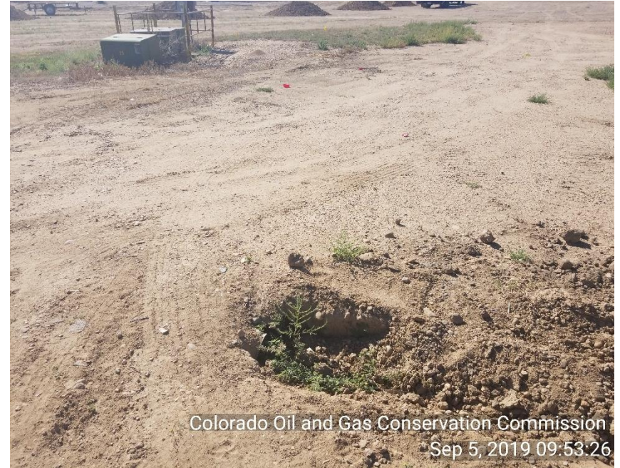
Photo 2 middle of culvert had been damaged prior to part of culvert being removed clearly see weeds growing in culvert.
