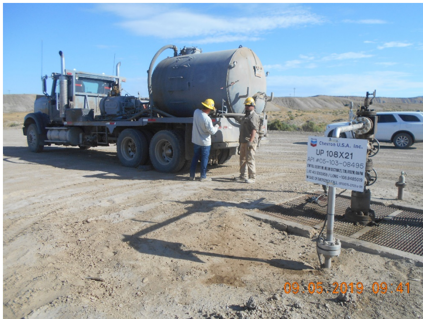
Injection wellhead with sign. Preparing for MIT.
