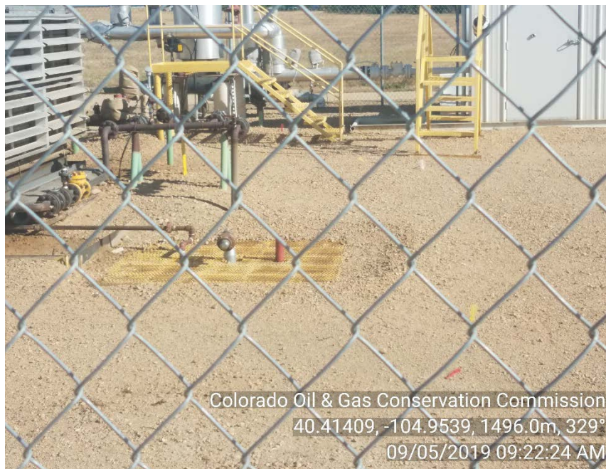
Unplacarded concrete vault
