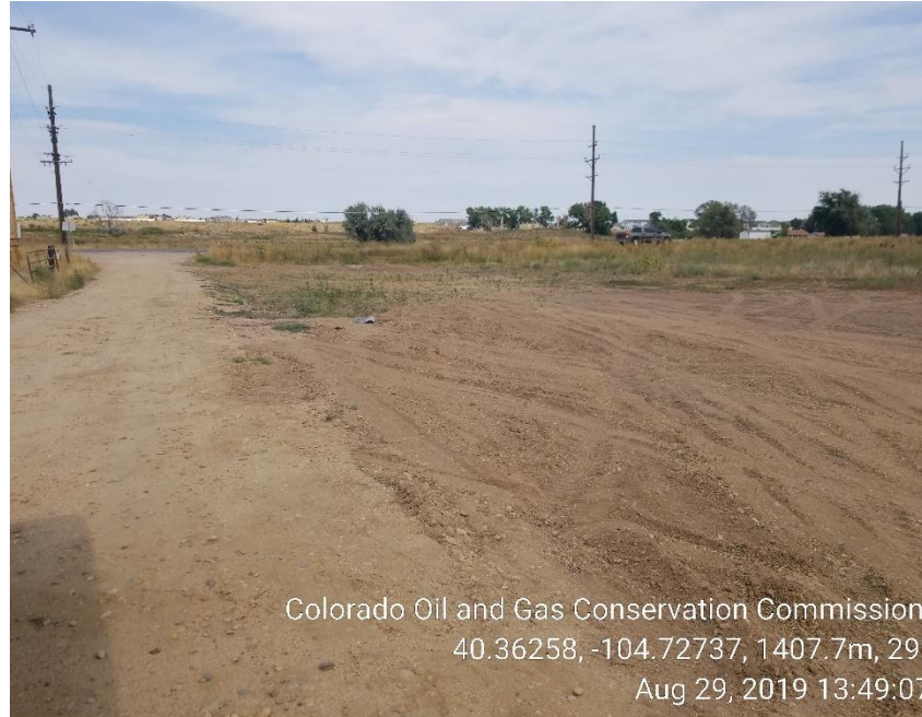
Photo 1: Gas meter house removed
