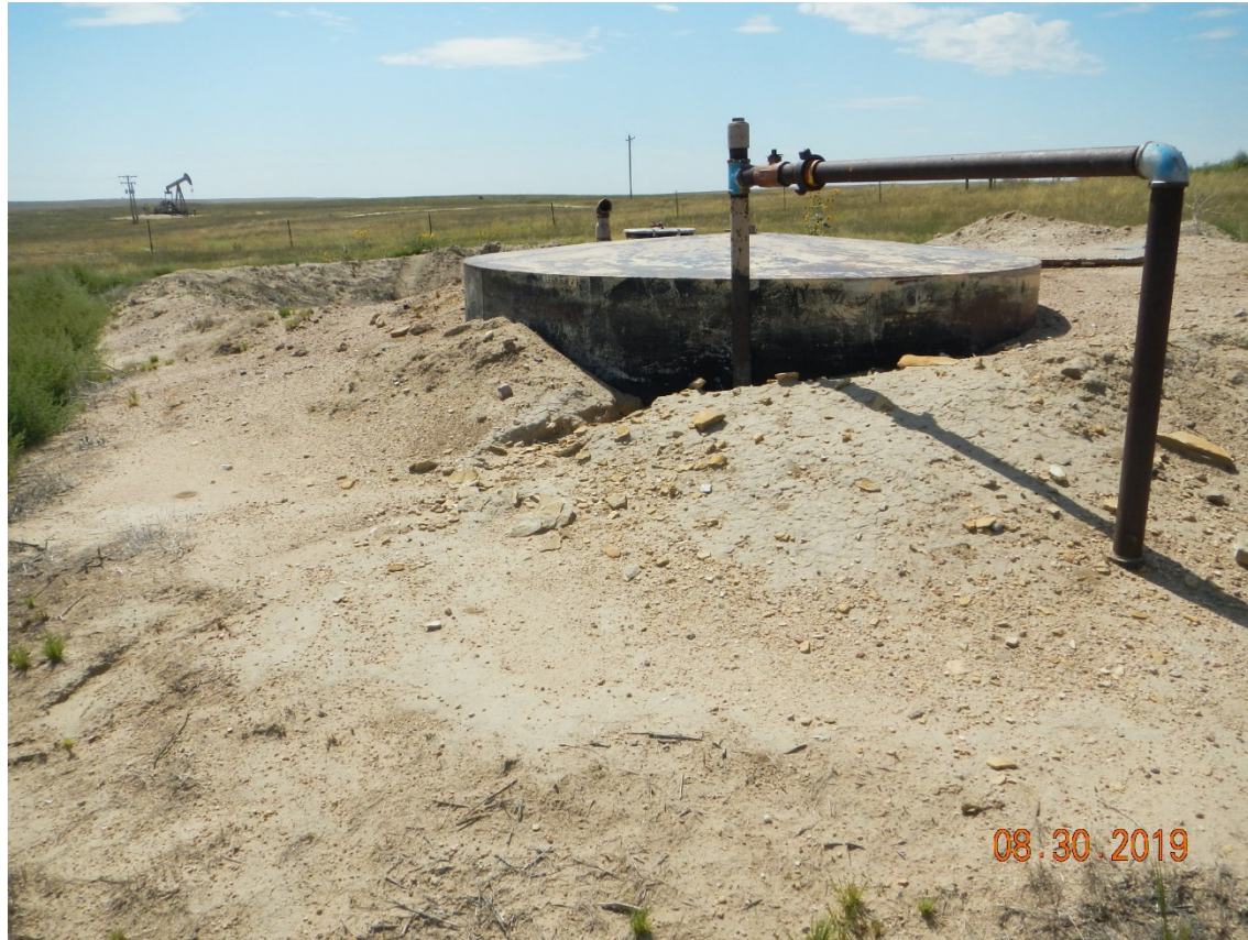
Photo # 1 – Partially buried oil slim tank with inadequate secondary containment on north side of Pit ID 112069
