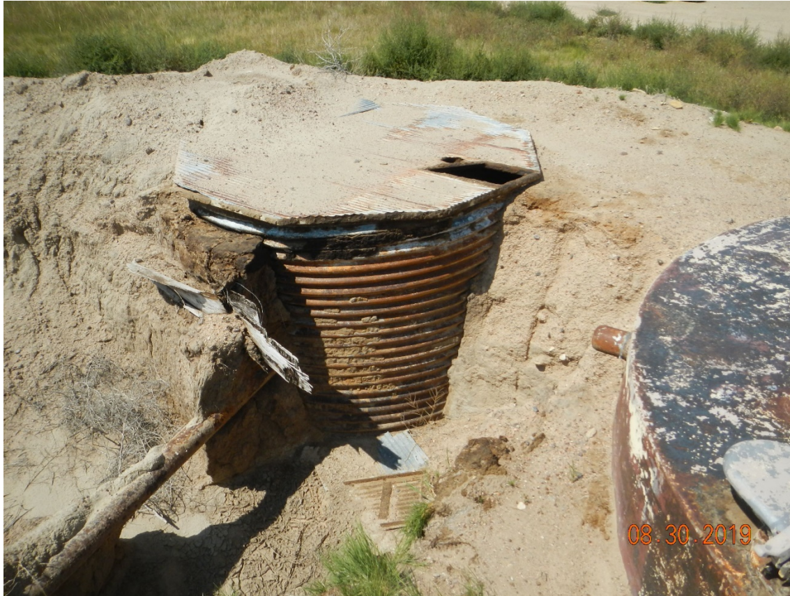
Photo # 2 – Culvert (tin horn) requiring closure under an approved eForm 27.
