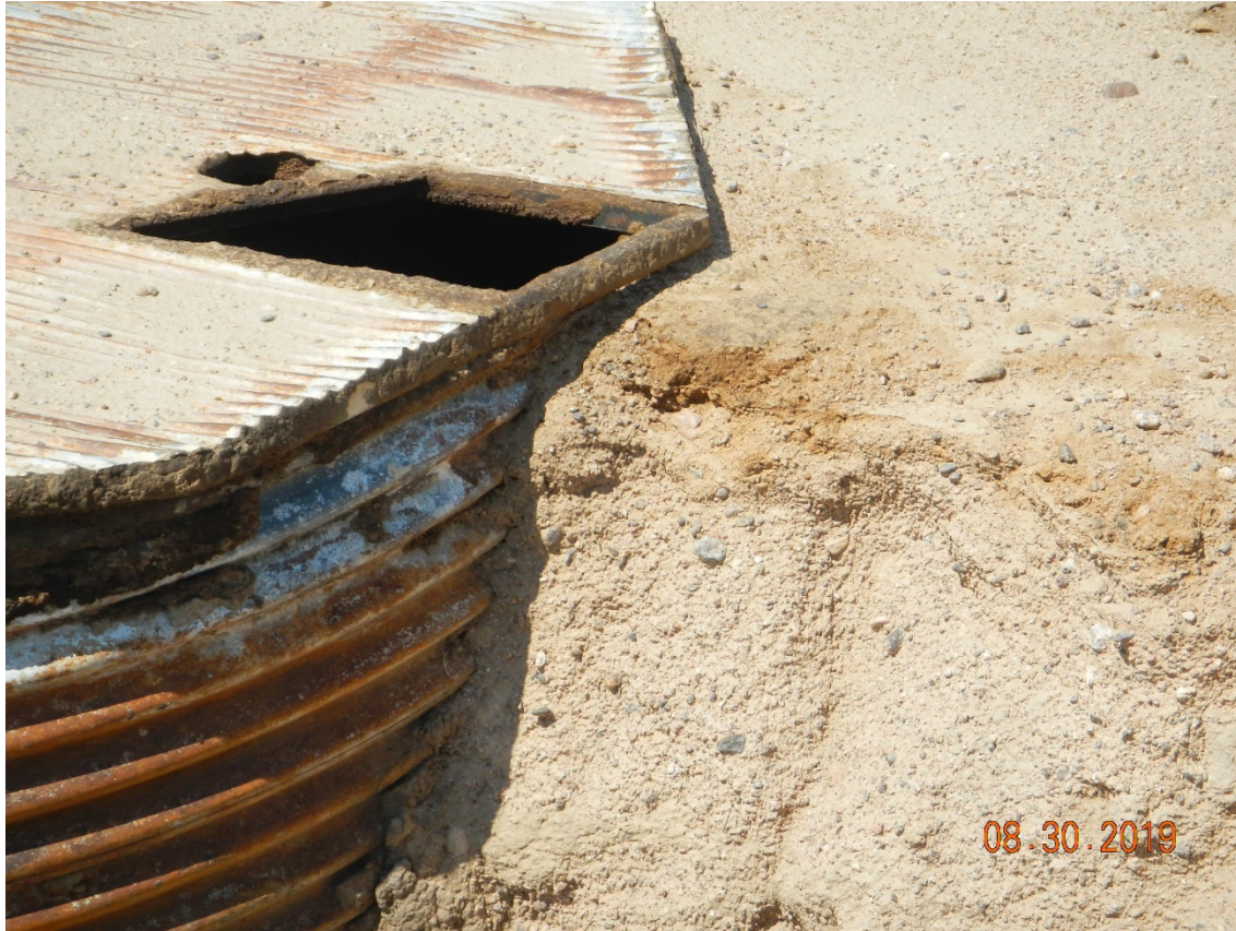
Photo # 4 – Petroleum impacted soil near culvert (tin horn) requiring closure under an approved eForm 27.
