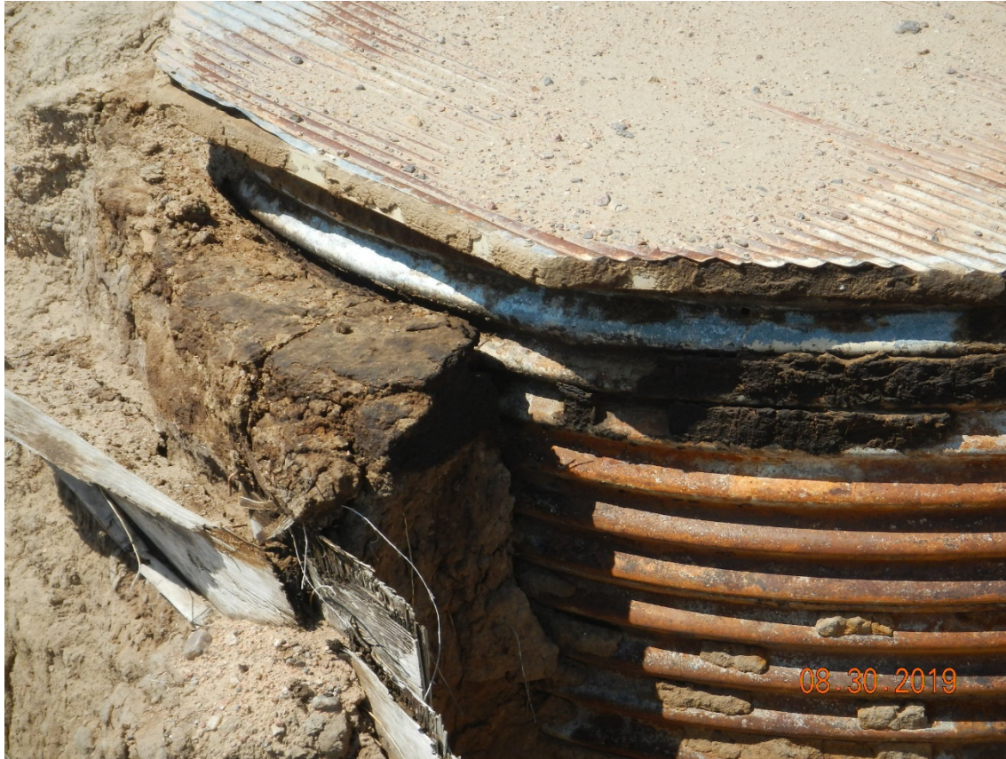
Photo # 3 – Petroleum impacted soil near culvert (tinhorn) requiring closure under an approved eForm 27.
