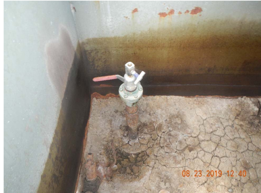
Photo 2. Photo of wellhead inside housing.
