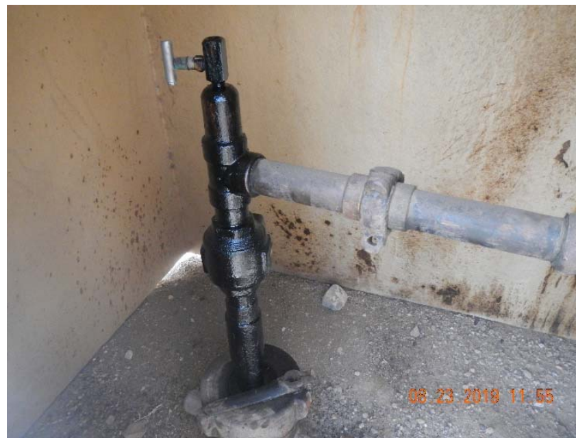
Photo 2. Photo of wellhead inside housing, stained soil at wellhead.
