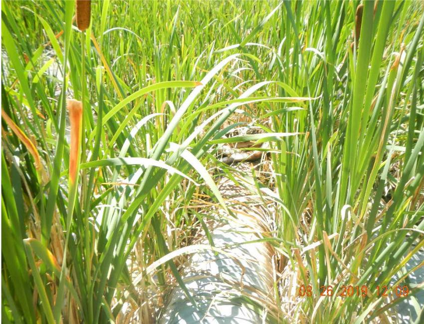
Photo #2 culverts that (passively) control level of water in upper pit, they flow to the lower pit
