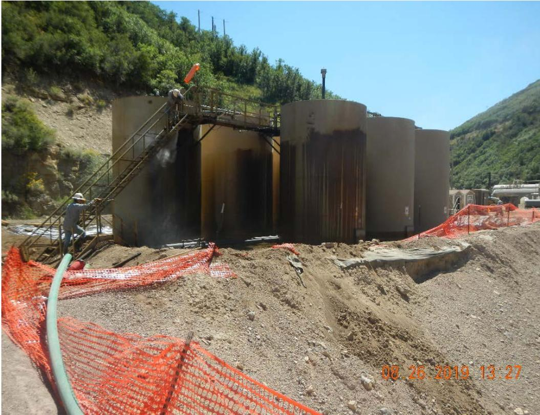
Photo #8 Tanks being cleaned. This was the source of spill. Pit is in process of closure is in foreground and right of photo.
