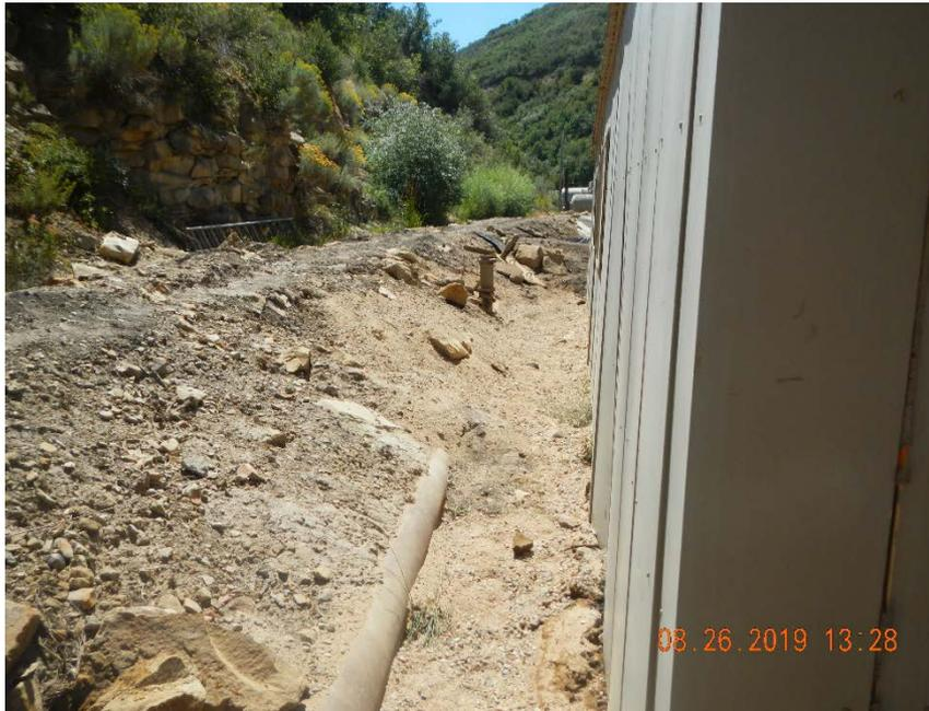
Photo #9. Injection Pump shed on right of photo. Photo is taken looking up grade (south), the tank battery (out of view) is behind the pump house. Spill path flowed between berm (at left of photo) and pump house. Fluid also went through the pump house.
