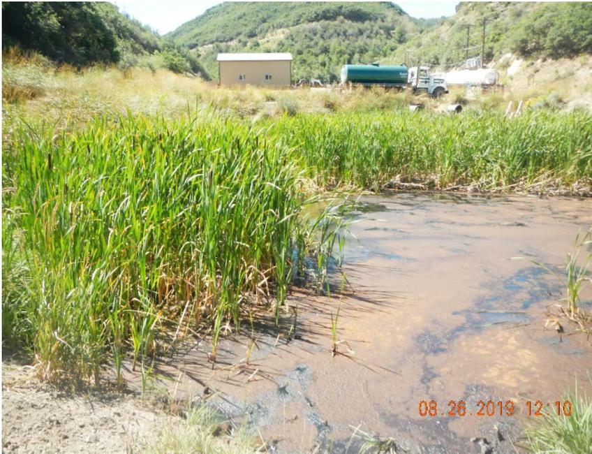
Photo #4 Upper pit. Photo taken standing on berm between pits. Oil on water in pit had “sphag sorb” applied, it shows up as brown on surface of water and was intended to absorb and encapsulate free oil on water surface.
