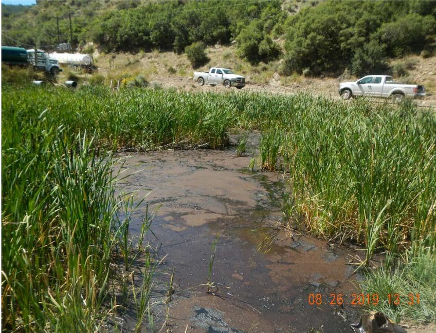
Photo #20 Photo of lower pit. Oil on water in pit had “sphag sorb” applied, it shows up as brown on surface of water and was intended to encapsulate free oil on water surface.
